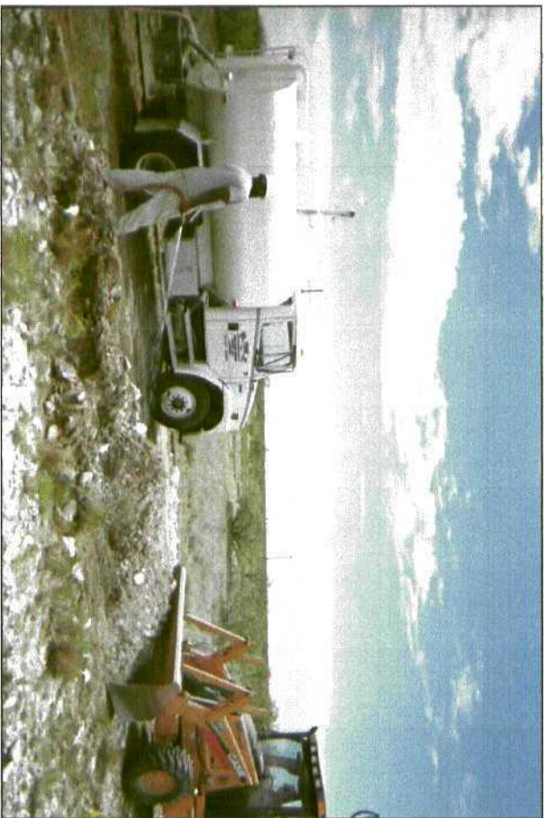
backfilling and compacting trench
