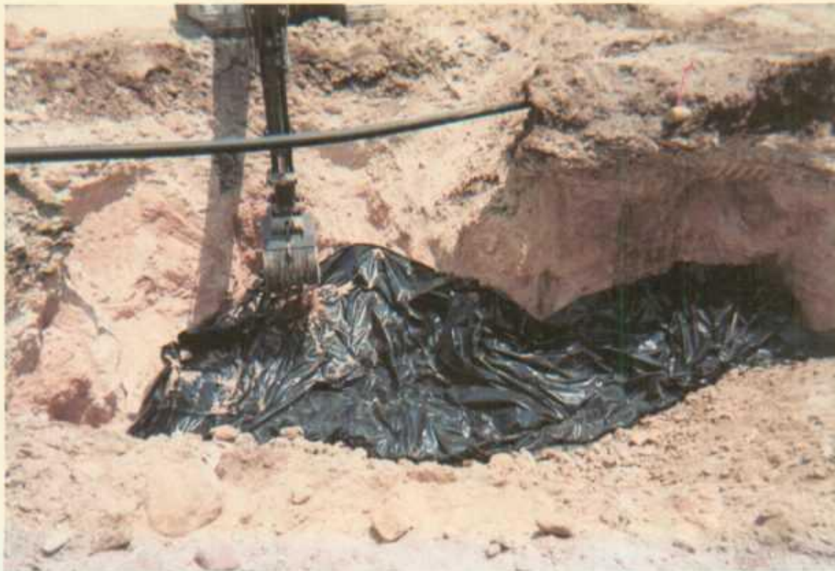
Installing Poly Liner
