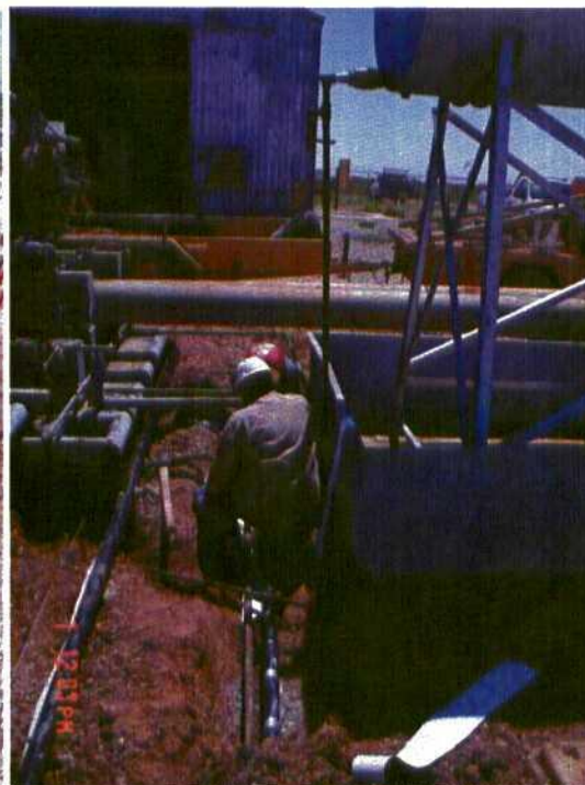
Photo 6. View to the east. Example of 20-mil polyethylene wrap on excavated pipe.
