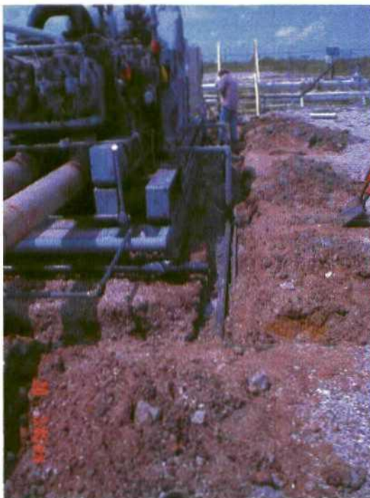
Photo 5. View to the north. Example of hand excavation on east side of Anderson Ranch compressor
