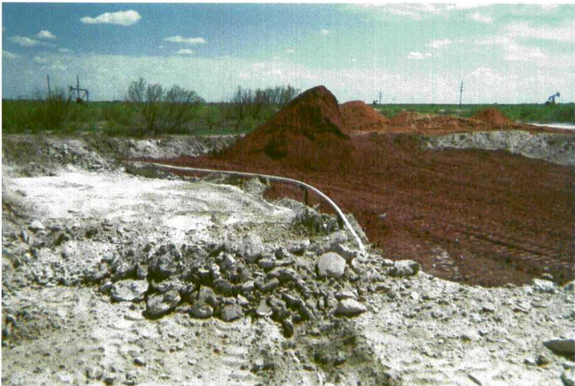
Justis J-25 Impact excavation; Installing clay liner
