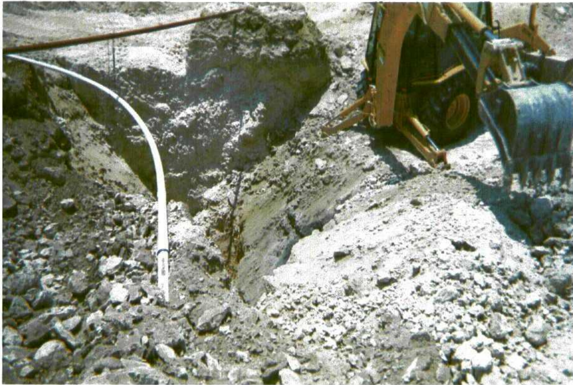
Justis J-25 Impact excavation; Installing clay liner
