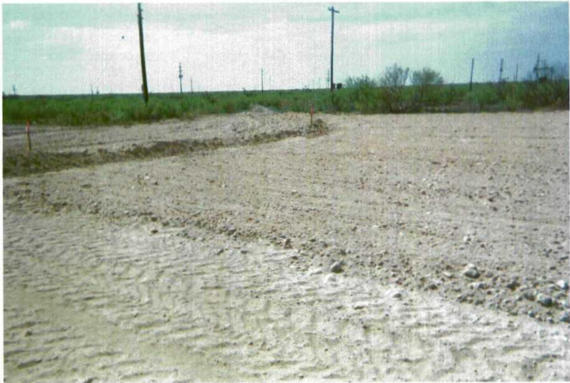
Justis J-25 Backfilled with blended soil.
