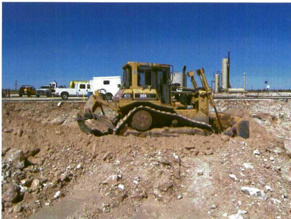
Figure 3: Placing south spoil pile in bottom of former pit
