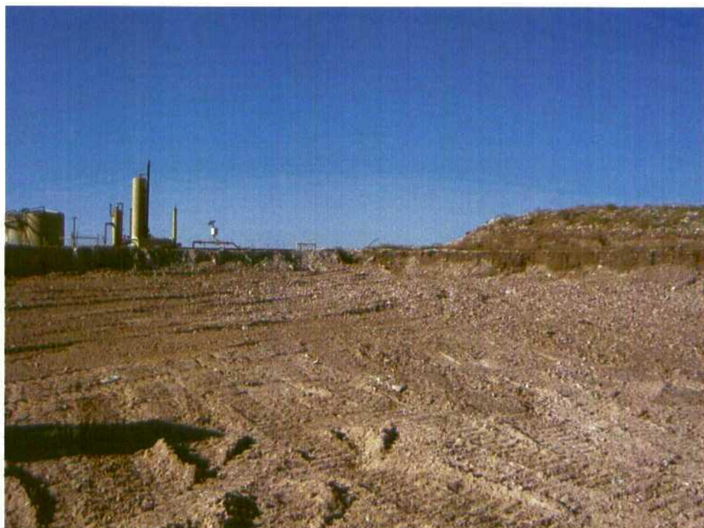
Figure 4: Placing coarse-grained east spoil pile material over south pile with northern soil pile in background. Layers show 5% slope.
