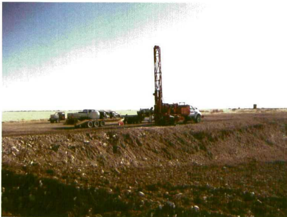
Figure 8: Drilling MW-4 prior to final grading
