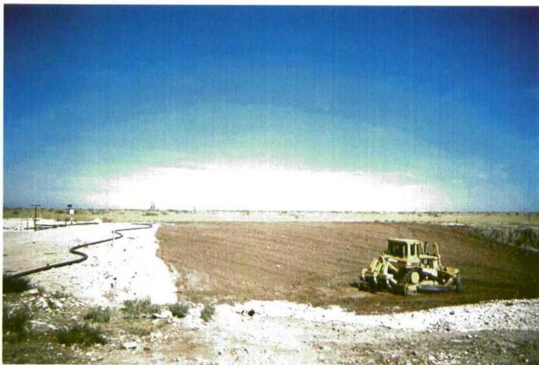
Figure 6: Grading to achieve 5% slope of topsoil cover
