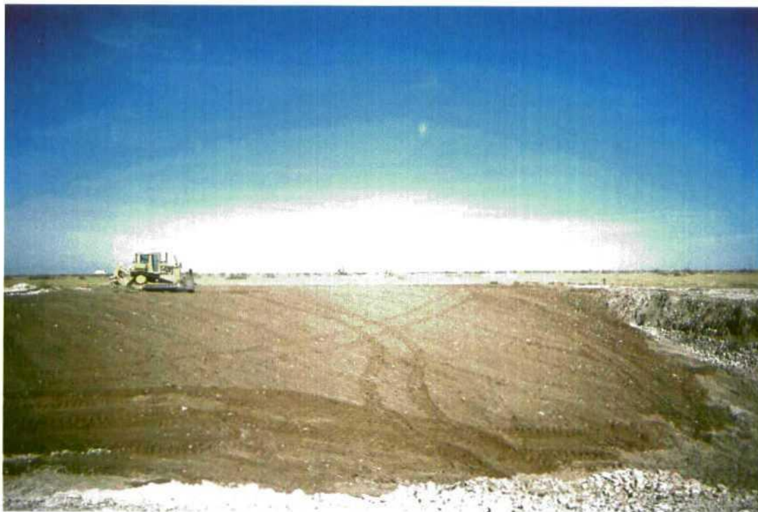
Figure 5: Placing topsoil from north pile over east spoil pile material
