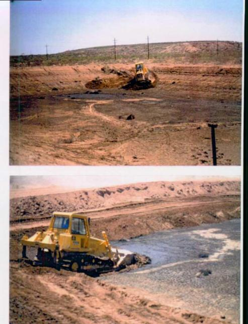
5. Excavation of heaviest section of sludge to 4 feet deep
