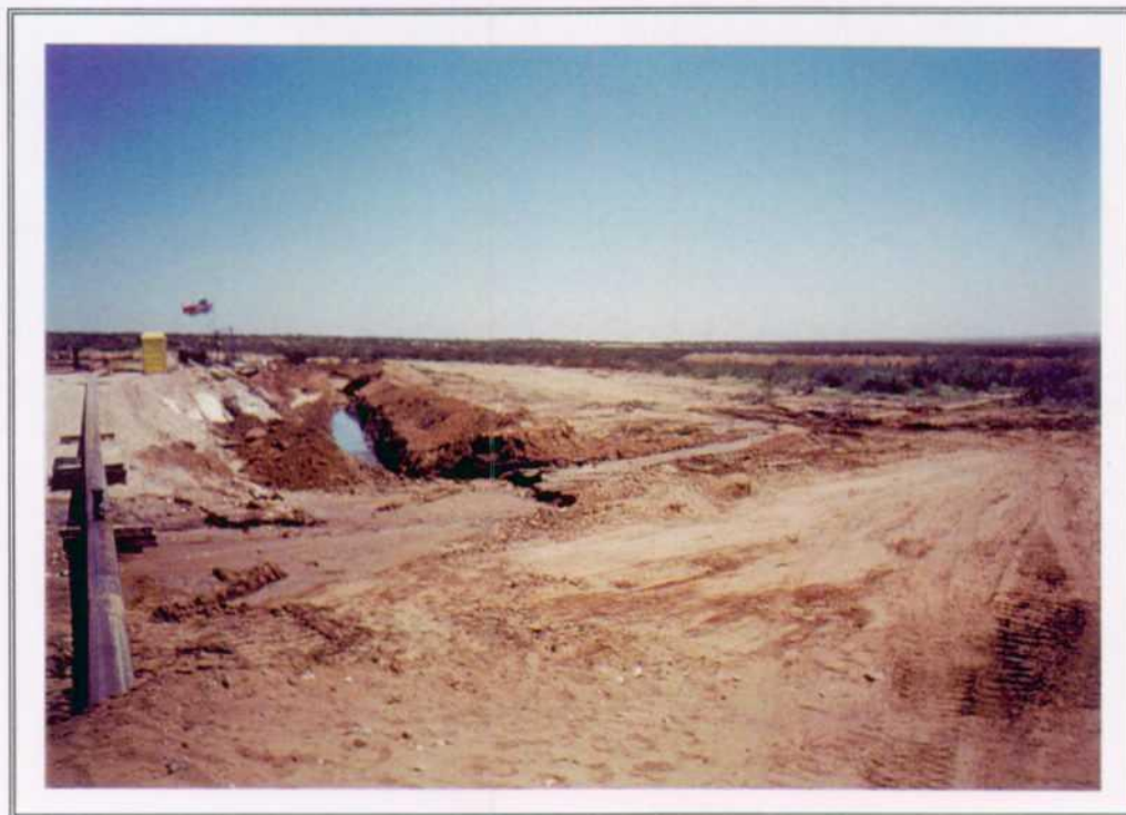
12. Trench #2 - fluids in trench during blowout.
