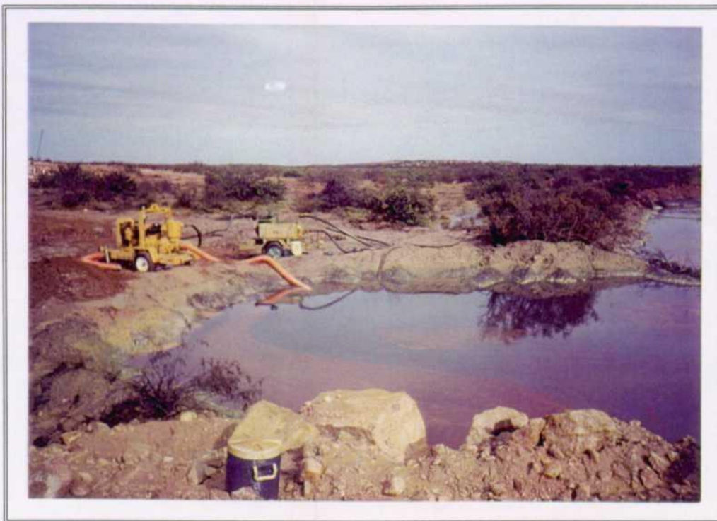
1. View of Trench #1 - pumping saltwater and oil to offsite pit.
