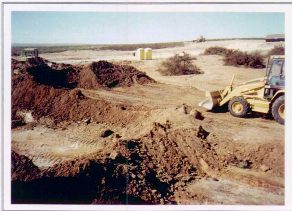
6. Trench #1 - soil excavation and remediation.
