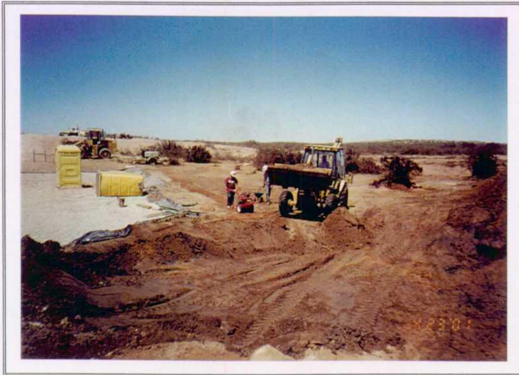
5. Trench #1 - soil excavation and remediation.
