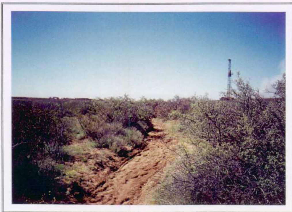
25. Dry Wash - soil remediation, after tilling.
