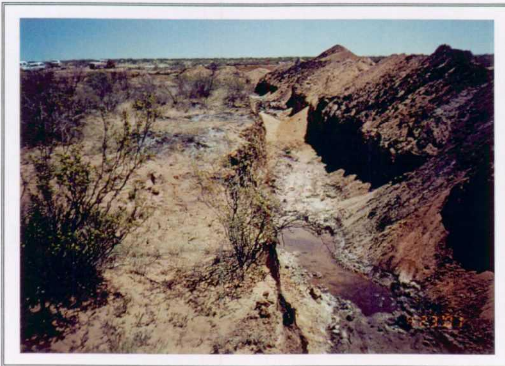
18. View of Trench #3 - fluids in trench during blowout.
