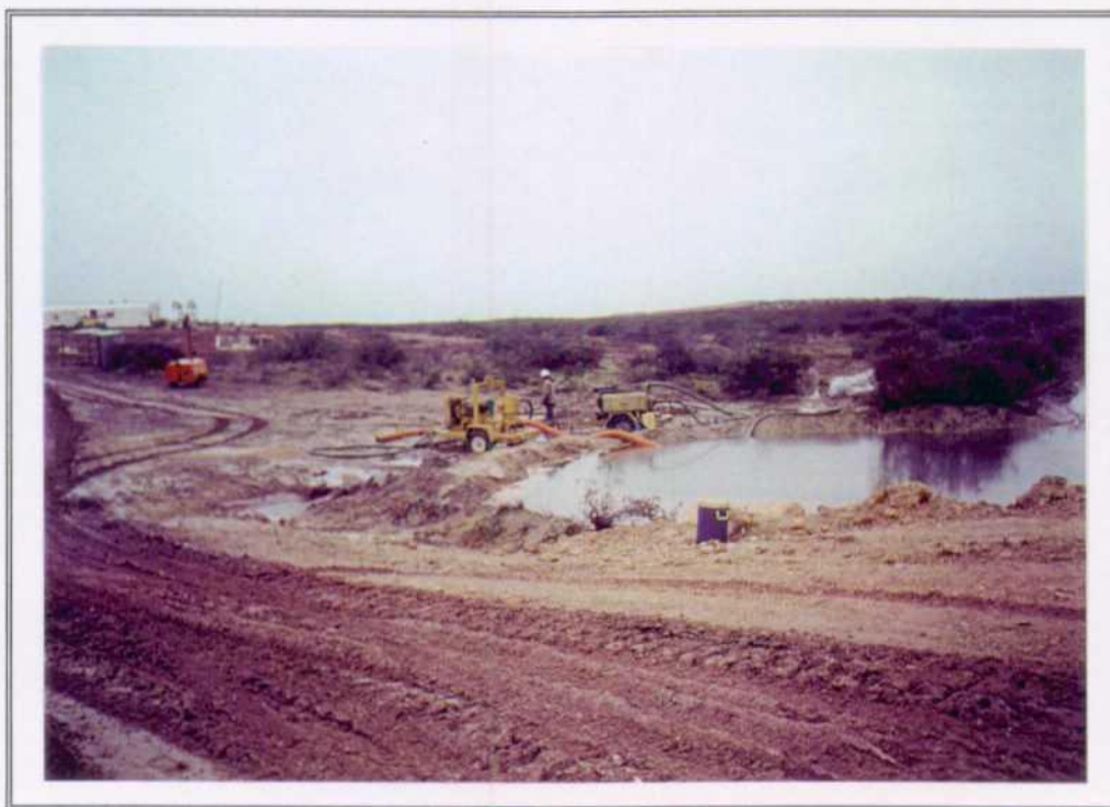
2. Trench #1 - pumping saltwater and oil to offsite pit.
