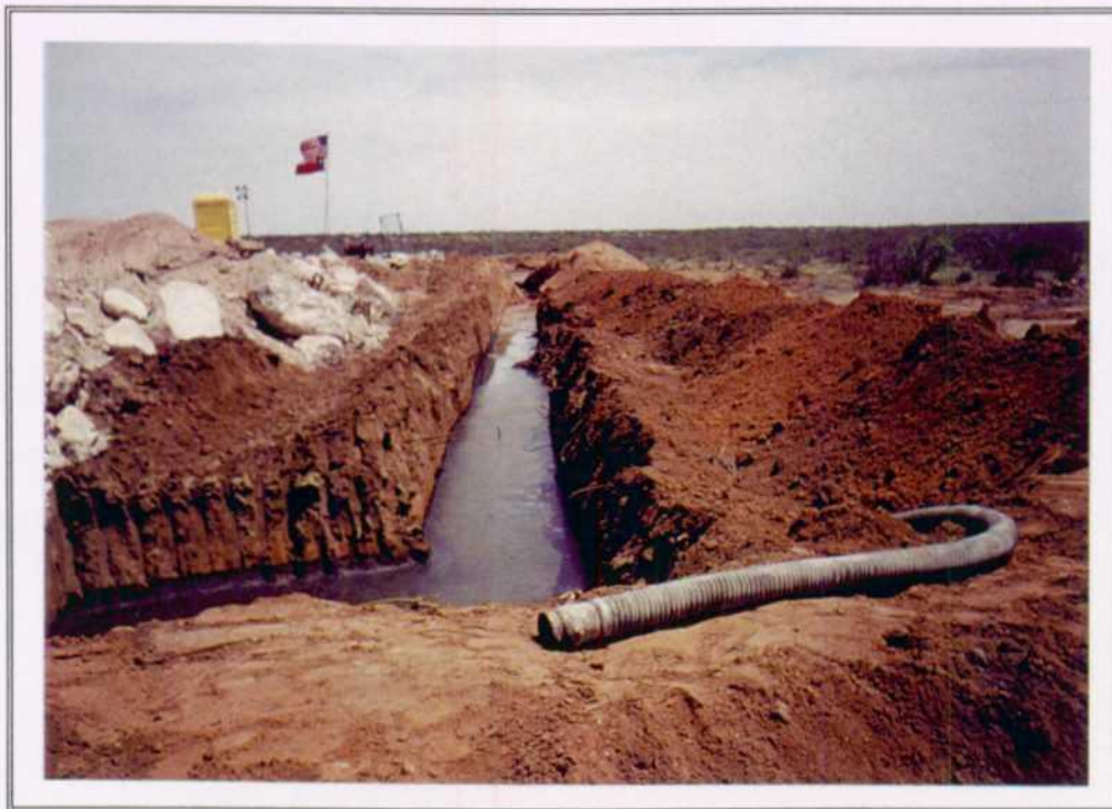
13. Trench #2 - fluids in trench during blowout.
