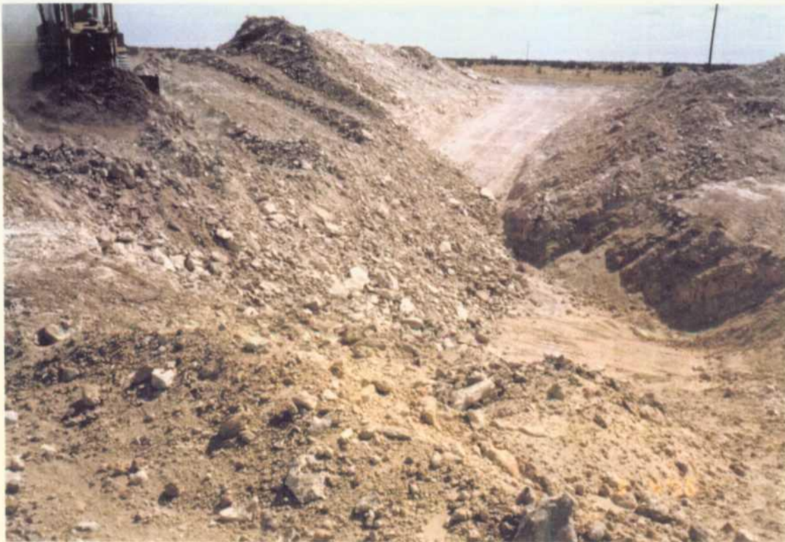
Backfill with clean soil.
