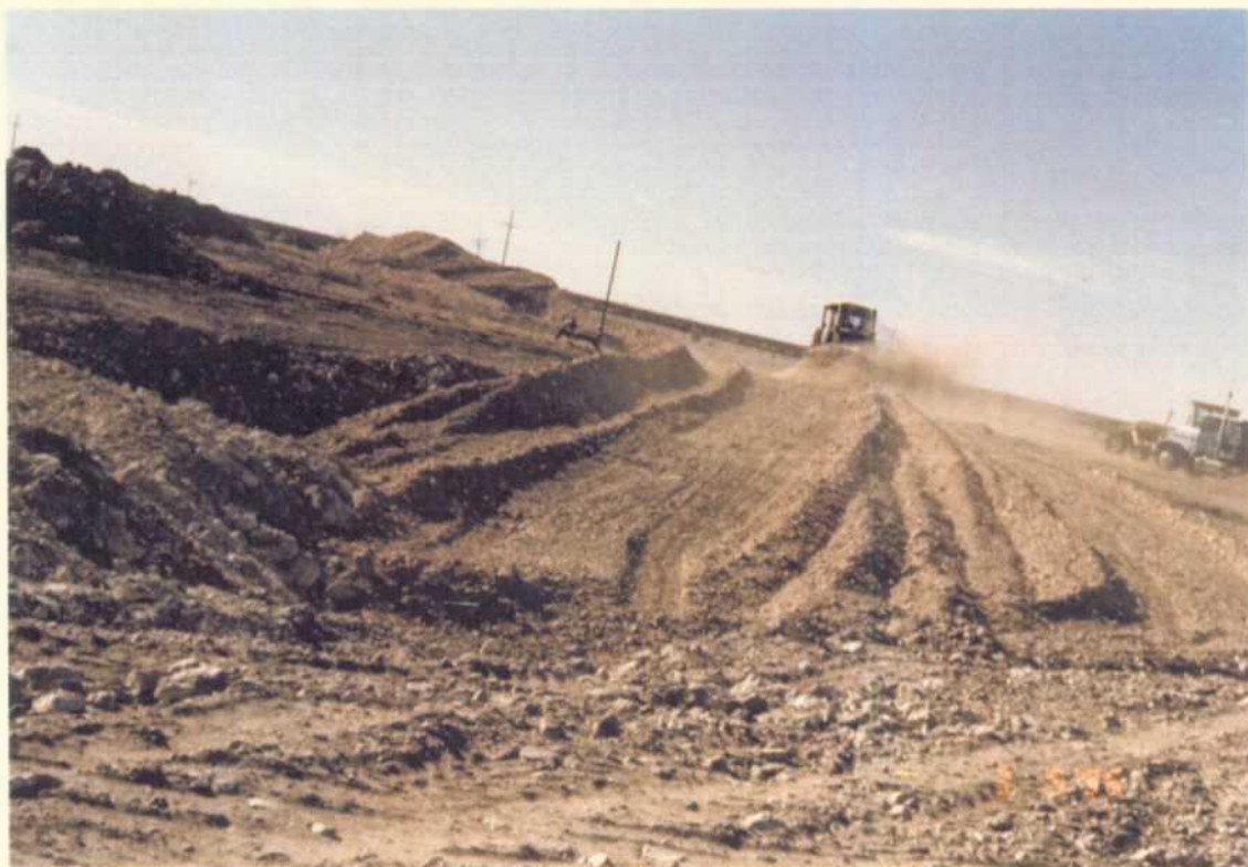
Clay cap in progress.
