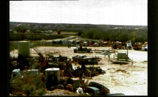
Overview of condensate tank, seperation unit and produced water pit at Amoco well GCU # 157E
