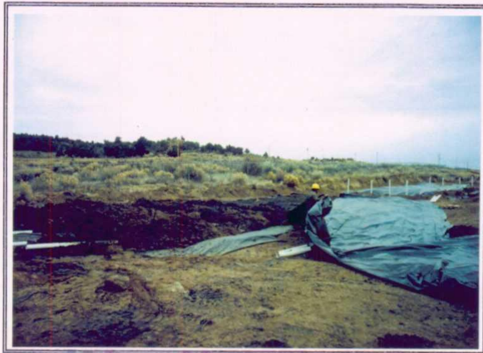
7. Northeast view of the treatment cells in the process of being covered with PVC liners. Treatment cell number one is in the background and has been covered with vertical vents in place.
