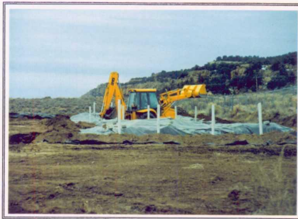
8. Northwest view with the treatment cells filled, covered and the covers in the process of being anchored. The salt cell can be seen in the background.
