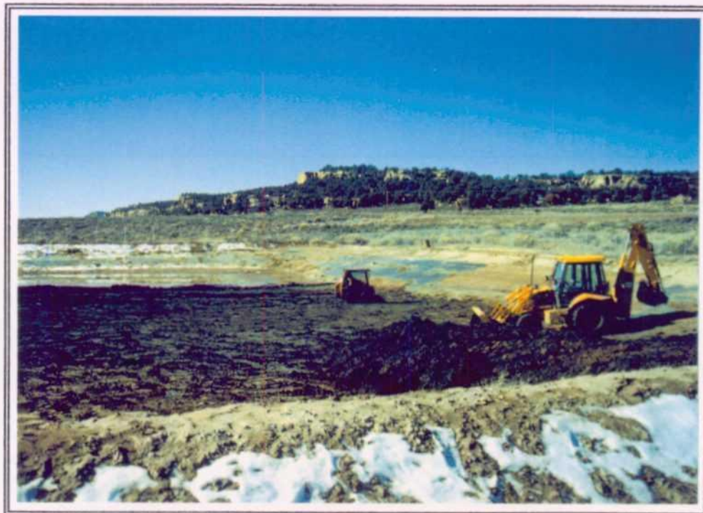
3. Treated sludge has been stockpiled in the corners of the cell and the liner is being prepared for removal and placement into a treatment cell.
