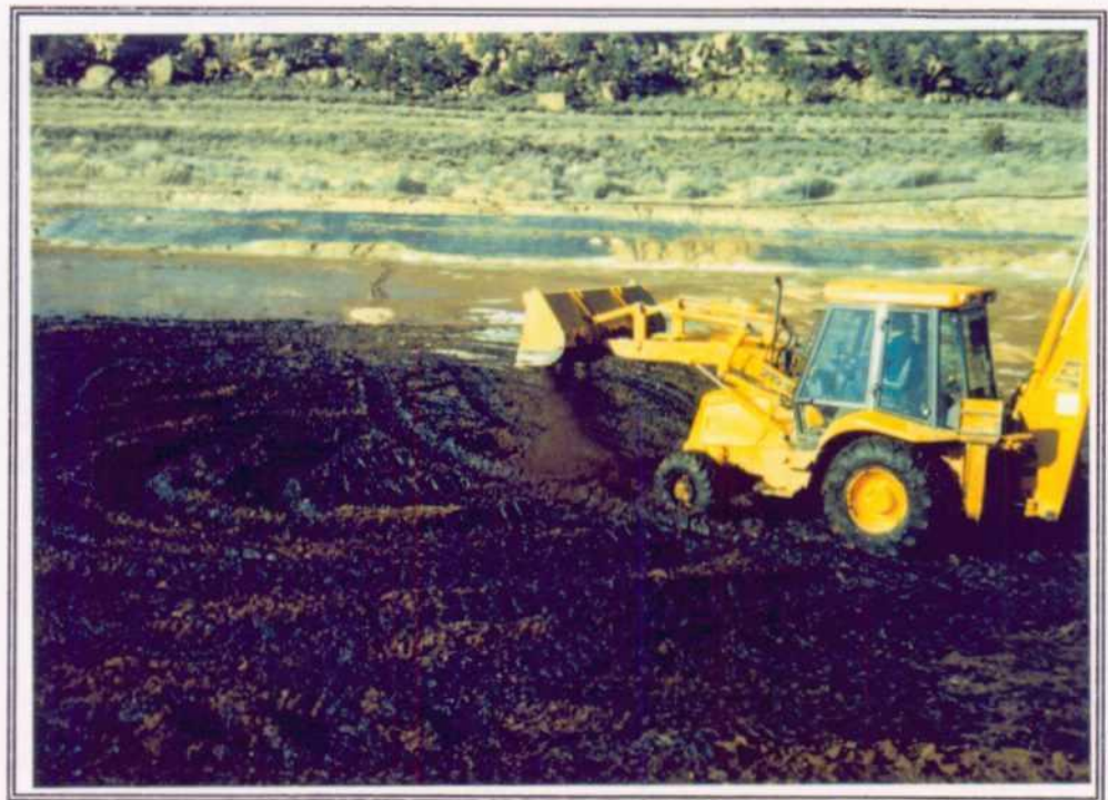
2. Mixing of compost material into the sludge before removal.
