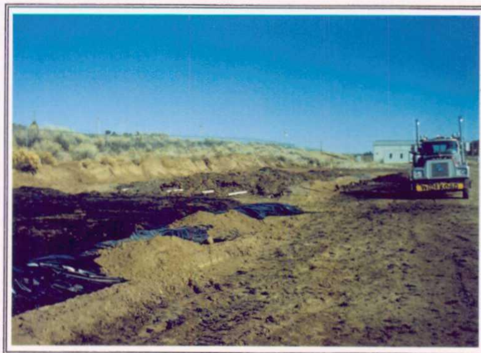
6. Northeast view of treatment cell number one after filling and awaiting covering. Treatment cell number two is in the foreground and still being filled.
