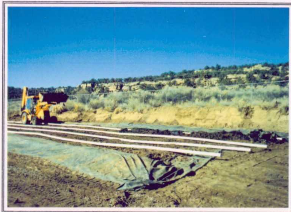
5. Constructed treatment cell with lower ventilation lines in place and the treated material being placed into the cell.
