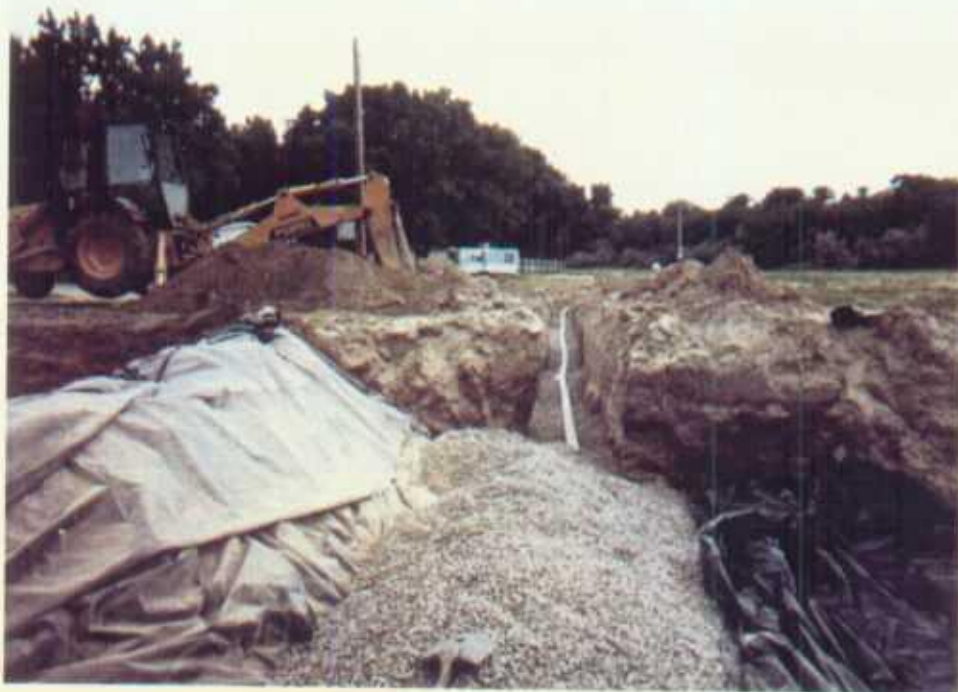
Vent pipe installed in trench near storage tank.
