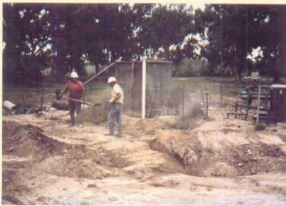
Production pit passive venting system is installed.
