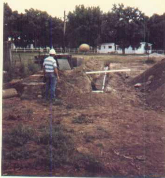
Vent pipe installed in trench near production pit.
