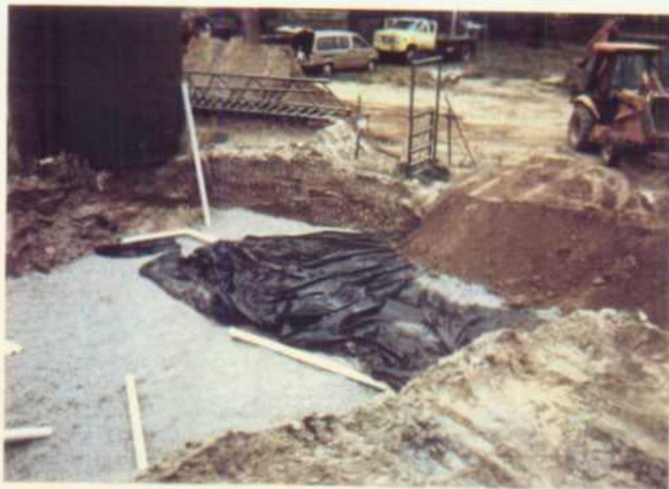
Gravel is installed in large excavation from level of groundwater to top of soil contamination. PVC is installed over gravel and clean dirt backfilled on PVC.
