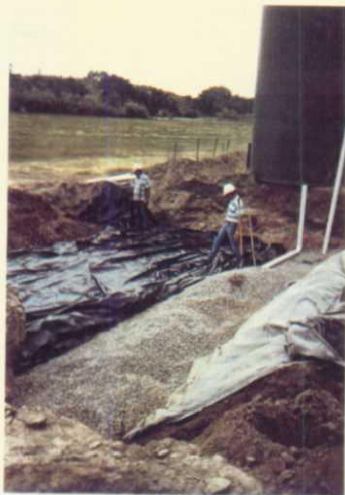
Vent pipe installed with mound of gravel over pipe. PVC sheeting is later folded over pipe.
