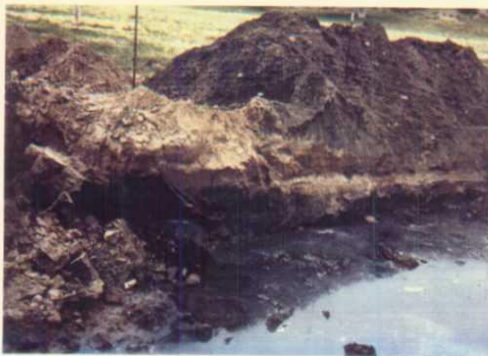
Photo looking west from storage tank. Note groundwater in excavation and thickness of contaminated soil.
