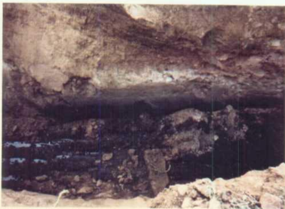
Photo by trench, 55 feet west of storage tank. Groundwater is present in trench. Note thickness of soil contamination is significantly less than near the tank.
