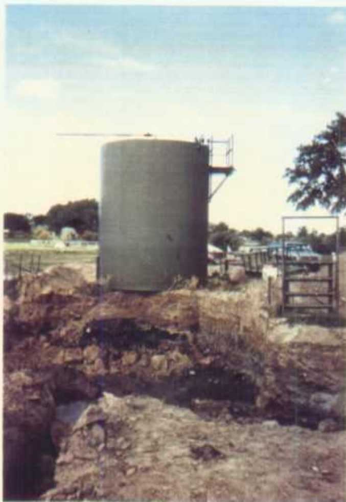
Photo looking east showing excavated area west of storage tank. Note discoloration of subsurface soils due to hydrocarbons. Groundwater is present in excavation.
