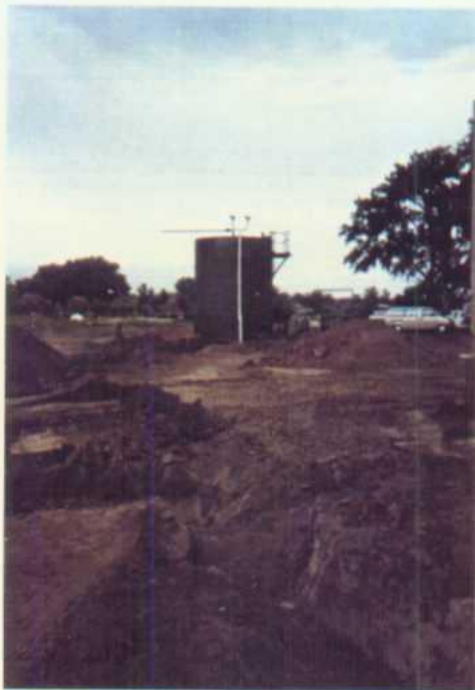
Storage tank passive system completely installed as surface restoration continues
