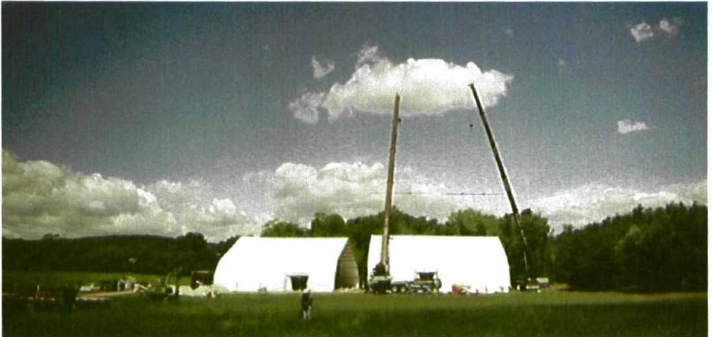
Construction Of Fabric Structure – Two Sections To Be Joined
