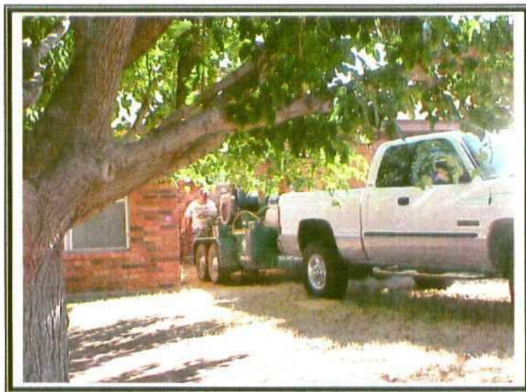
19) Portable rig being moved into position in between houses.
