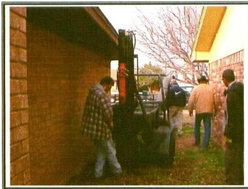
Soil Sampling – Borehole # 1506-02
