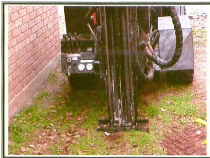
Soil Sampling - Borehole # 1506-04
