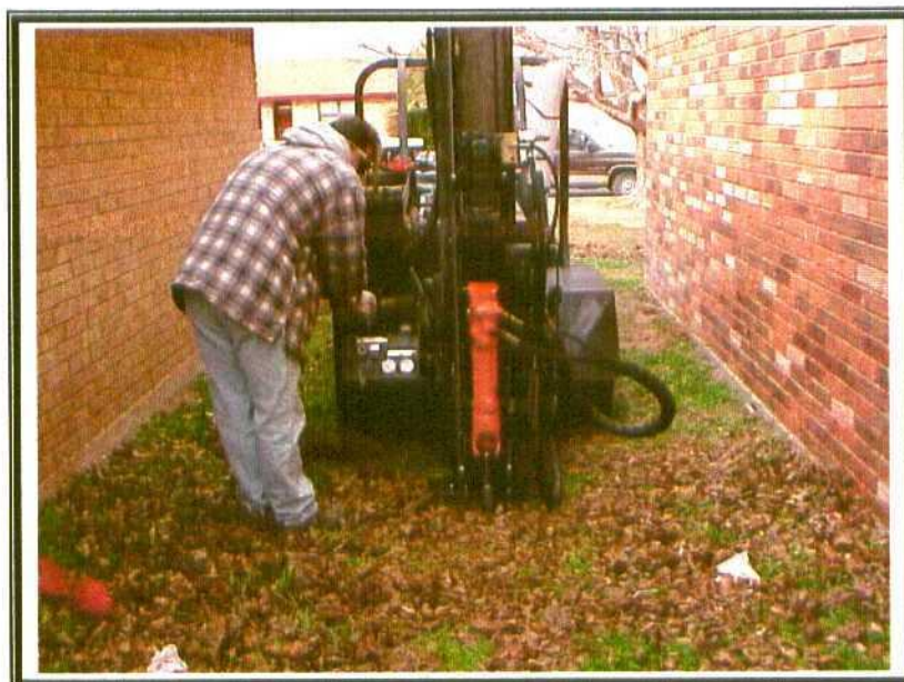
Soil Sampling - Borehole # 1506-03
