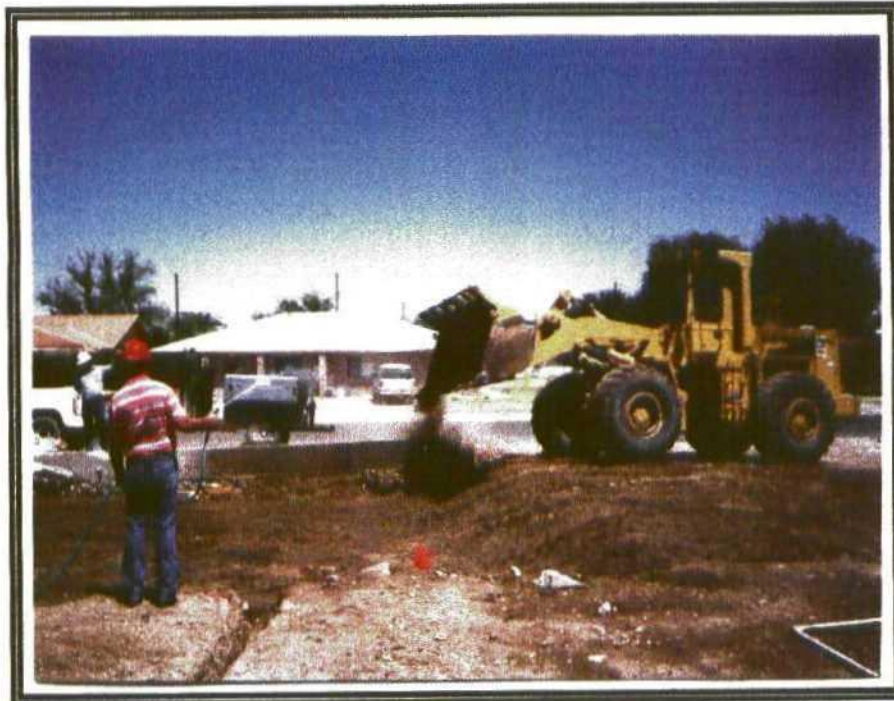
Foundation Removal
