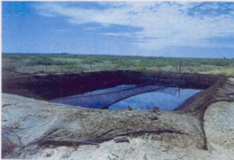
Photo 1: Inex Tank Battery unlined disposal pit prior to Yates' acquisition of the site.
