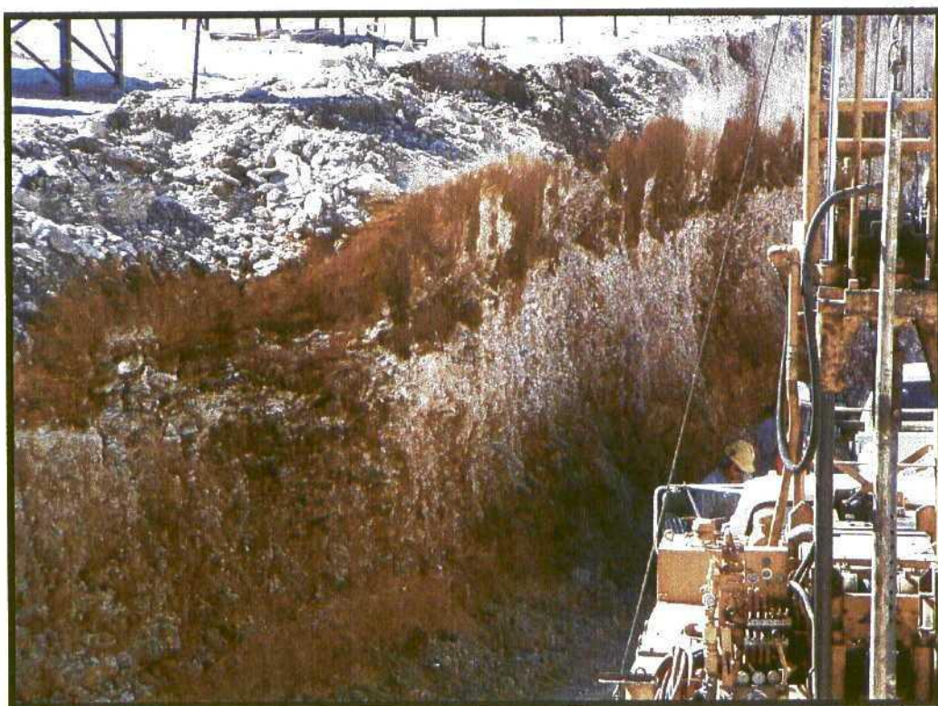
Installation of temporary recovery wells at the Monument pipeline release site, November 13, 2002 The pipeline was located adjacent to the base of the hydrocarbon stained soil on the left wall.
