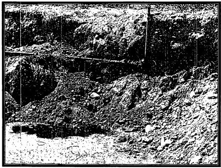
Photo 9: Additional Contamination from a Pipe Leak under the Separator
