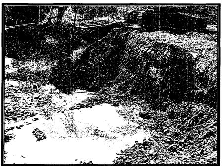
Photo 8: Removing Contaminated Soil on South Side of Excavation
