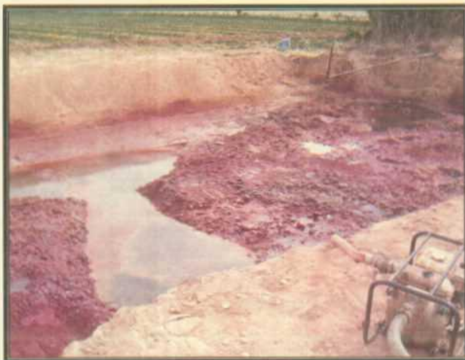
Photo 12: Final Treatment with Potassium Permanganate Solution
