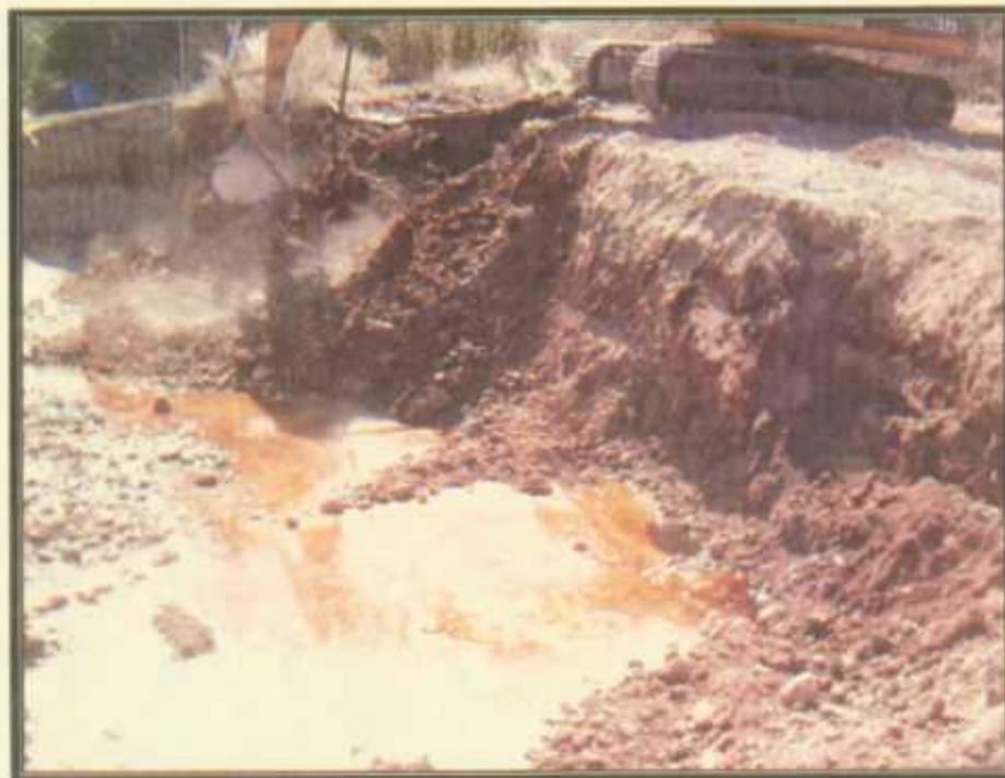
Photo 8: Removing Contaminated Soil on South Side of Excavation
