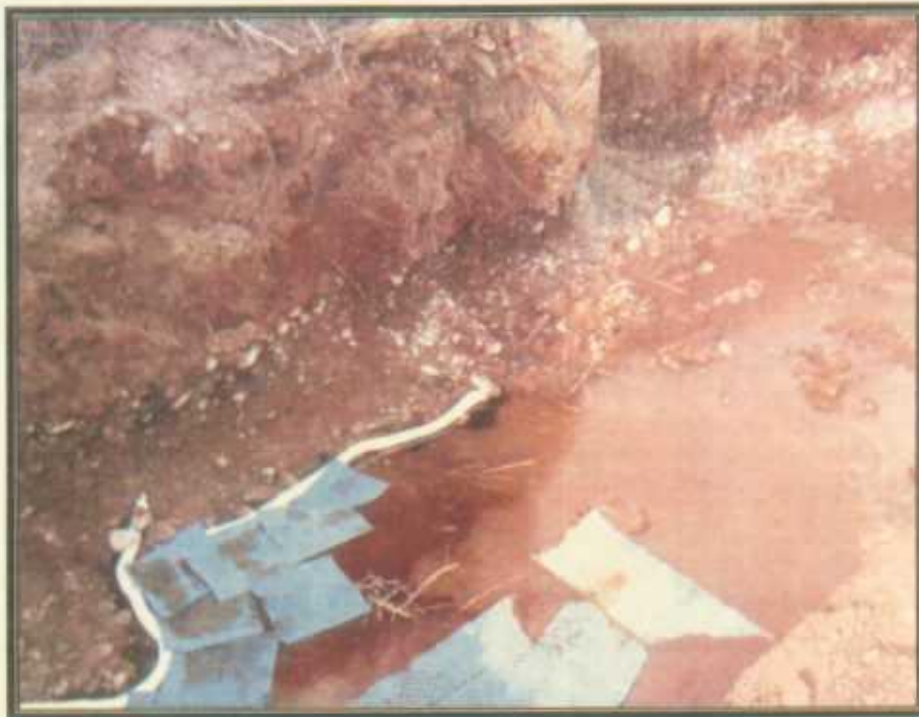
Photo 7: Absorbent Devices Placed to Prevent Further Leeching of Contamination into Groundwater
