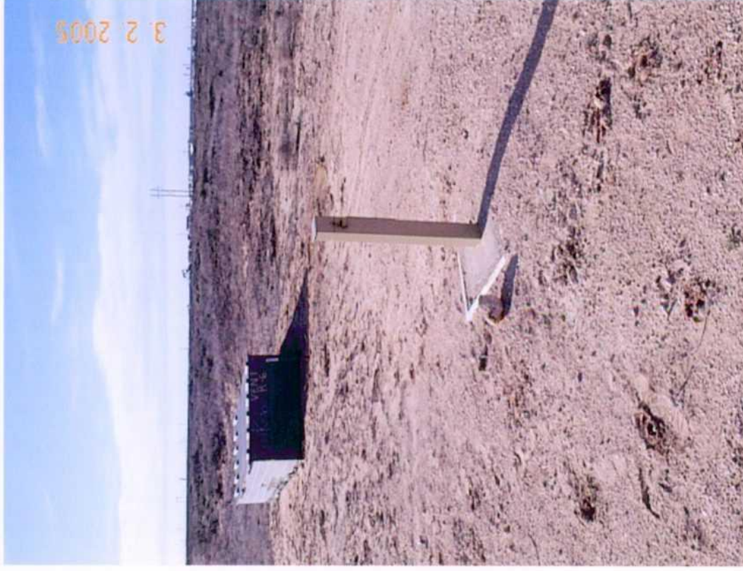
View of K-6 vent junction box (in background) after upgrade to lined watertight plastic junction box. Monitoring Well (MW-1) is shown in foreground.
