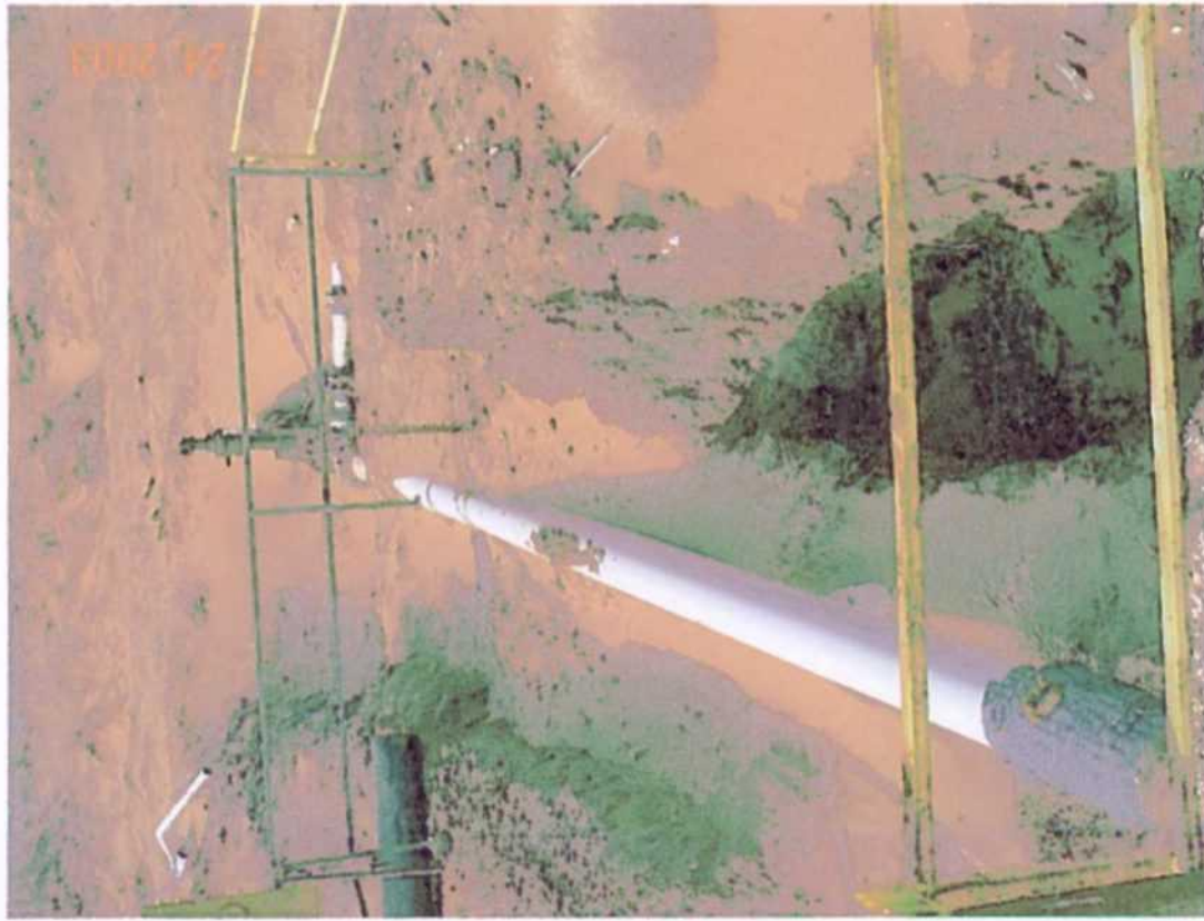
View of K-6 vent site after pipeline upgrade from 10-inch A/C to 6-inch PVC.
