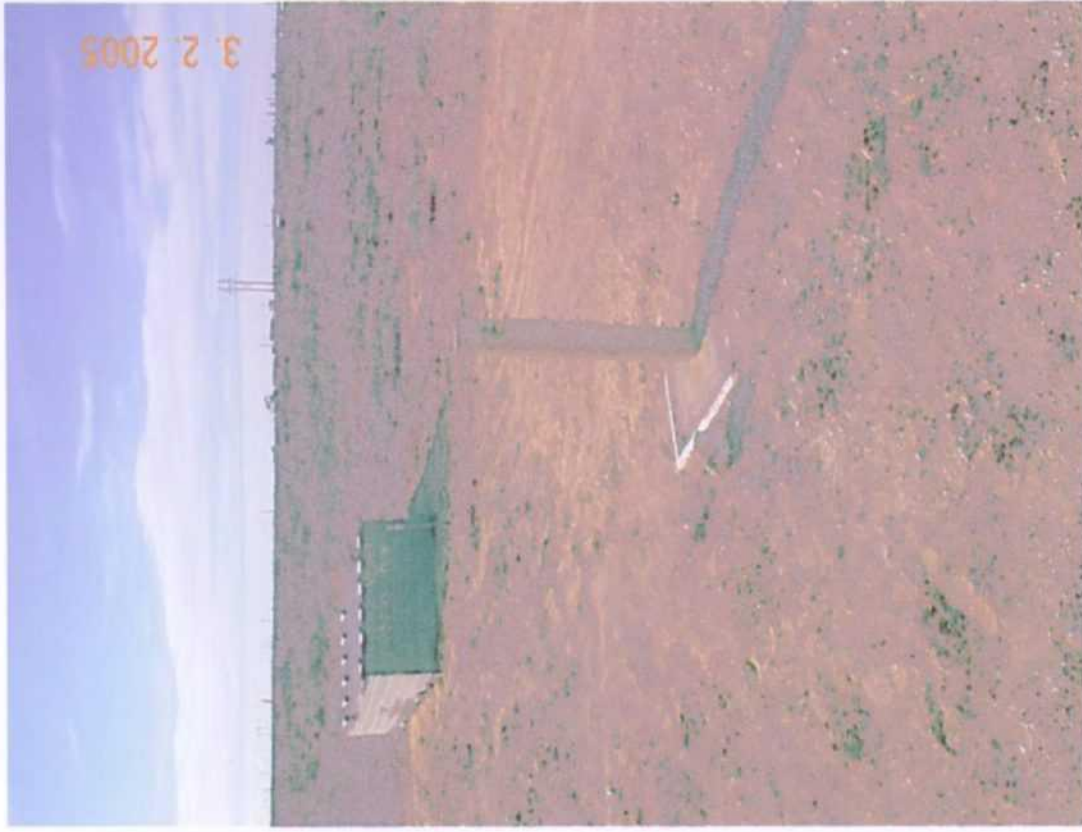
View of K-6 vent junction box site after upgrade to lined watertight plastic junction box.
