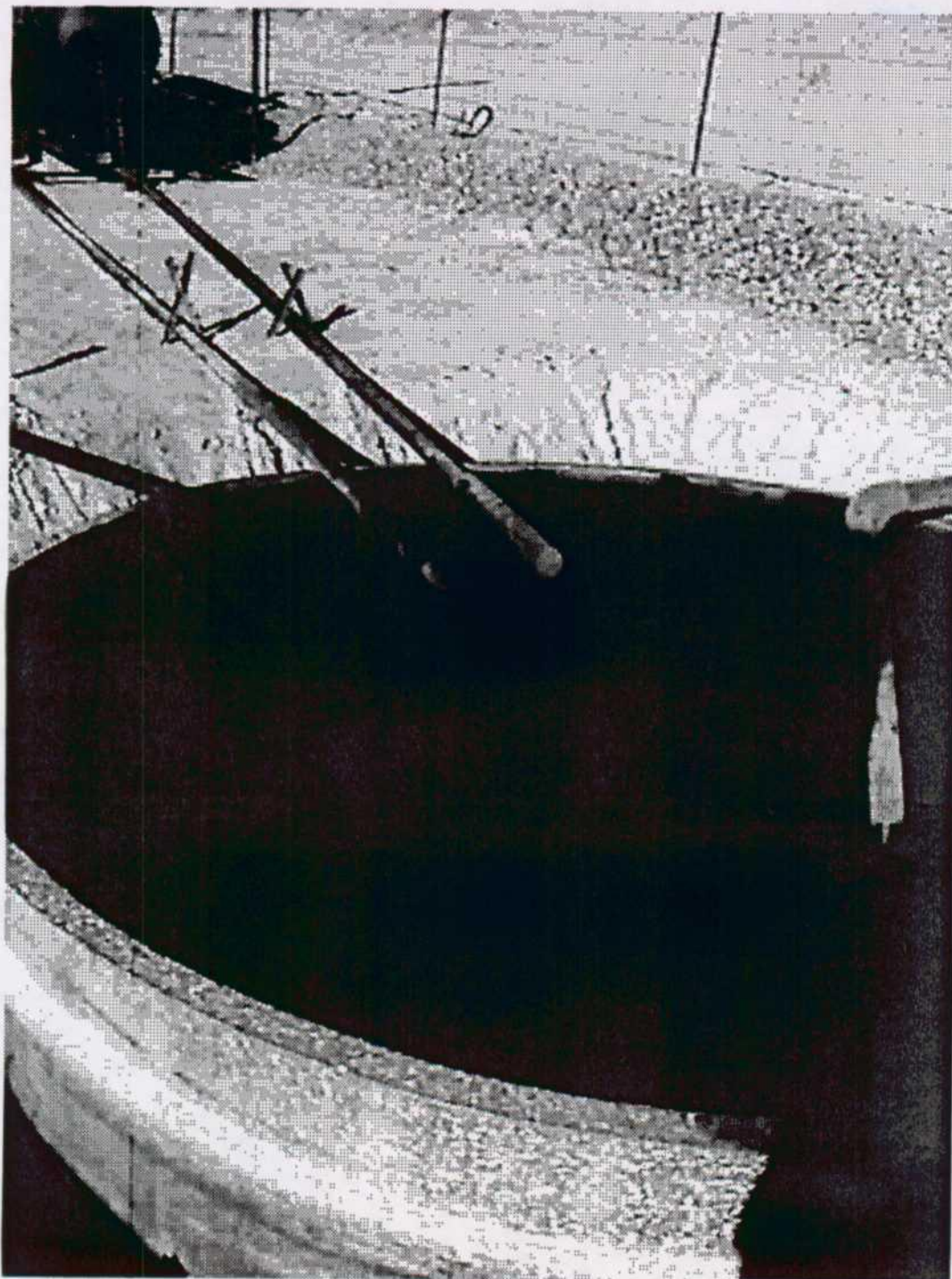
Burlington open tank at Hampton 4M – standing water w/minor amounts of product; at the time this picture was taken, there was no discharge to Burlington's open or closed tank, but Williams' dehydrator was being by-passed and free product was going to Williams' tank (March 1, 1999)
