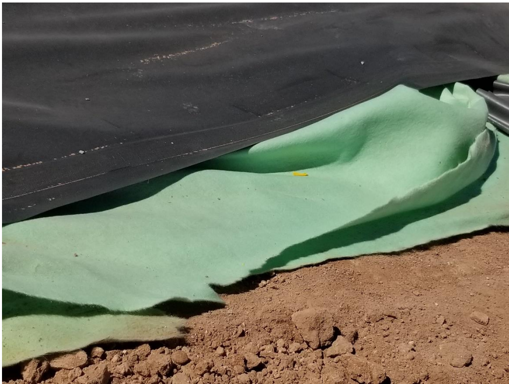
Photo 2: View of felt layer beneath first liner
