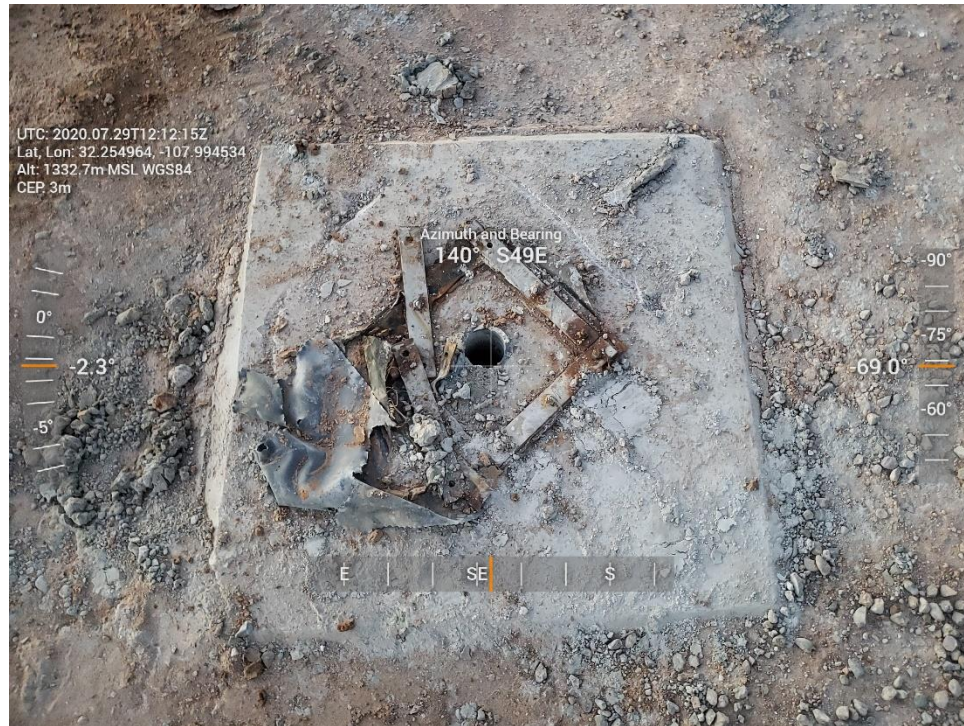
Photo 7: Excavation of concrete discharge vent
