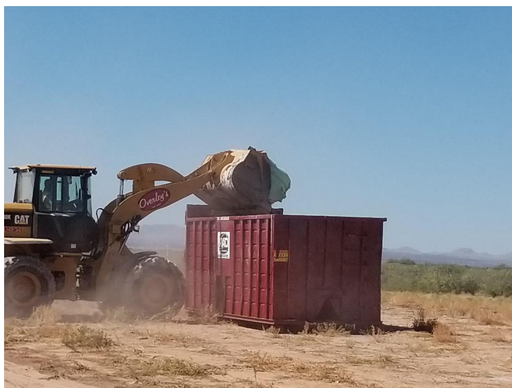
Photo 4: Liner material getting loaded into roll-offs
