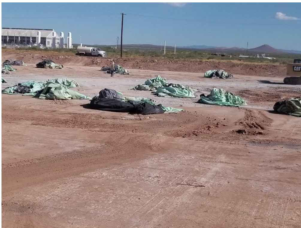
Photo 3: Liner material bundled for transport to roll-off
