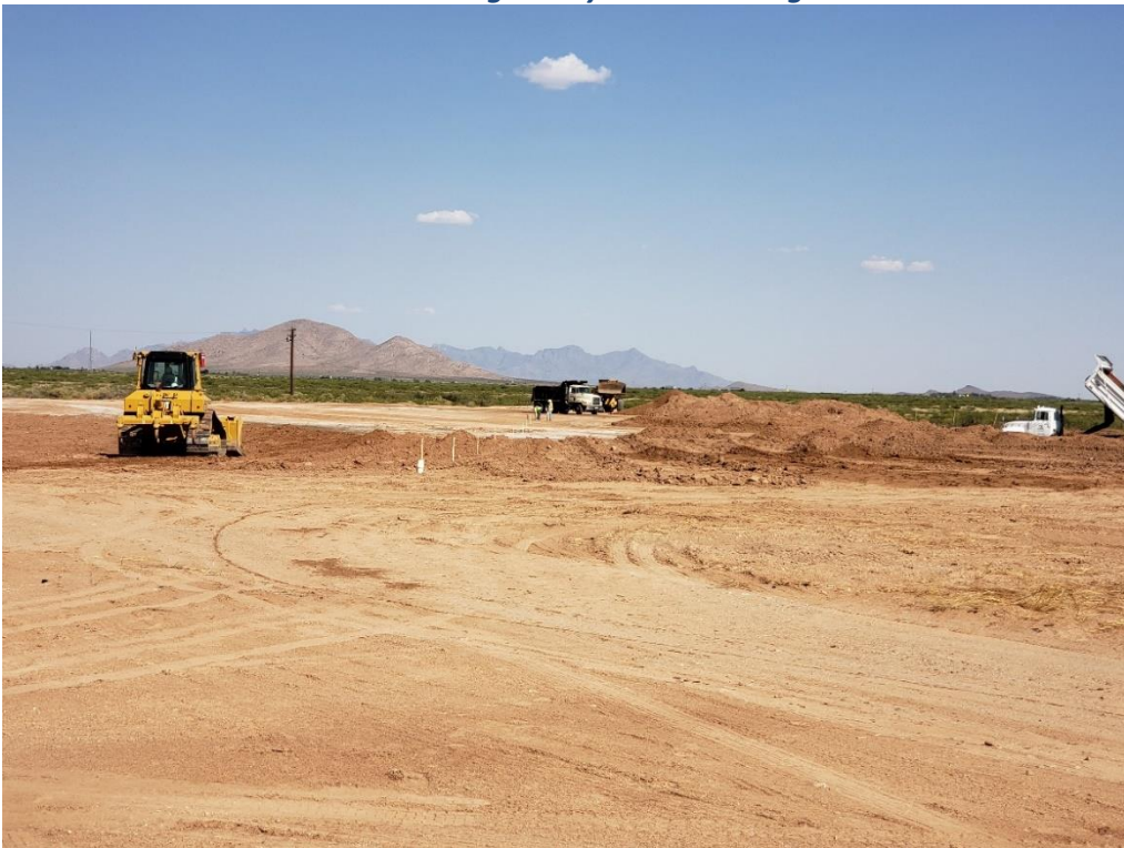
Photo 12: Import soil unloaded for backfill
