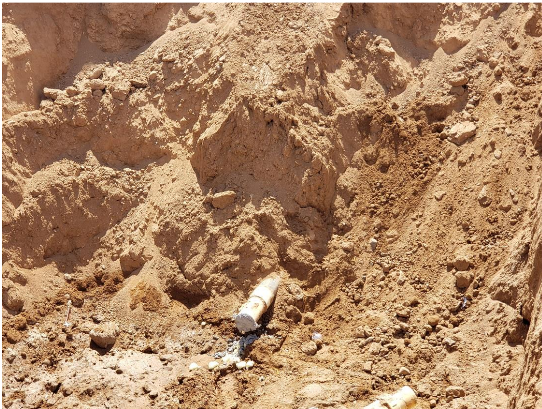
Photo 8: Drain line cut and plugged with concrete
