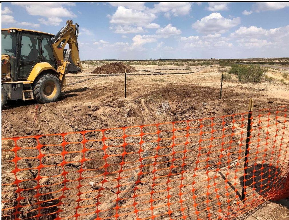
PHOTO 1: View of release origin, facing northeast. 8/14/2019
