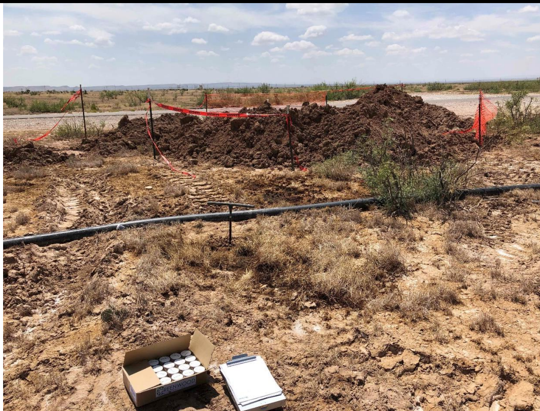
PHOTO 5: View of HA-6, facing south. 8/14/2019
