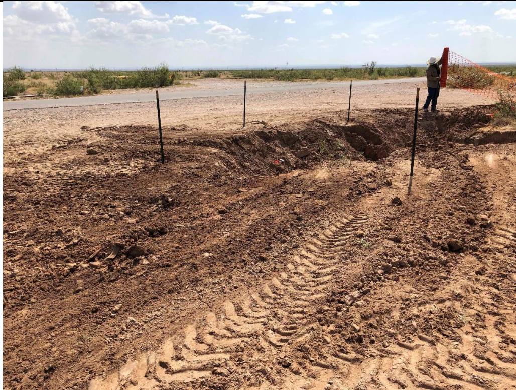
PHOTO 2: View of site securing, facing west. 8/14/2019
