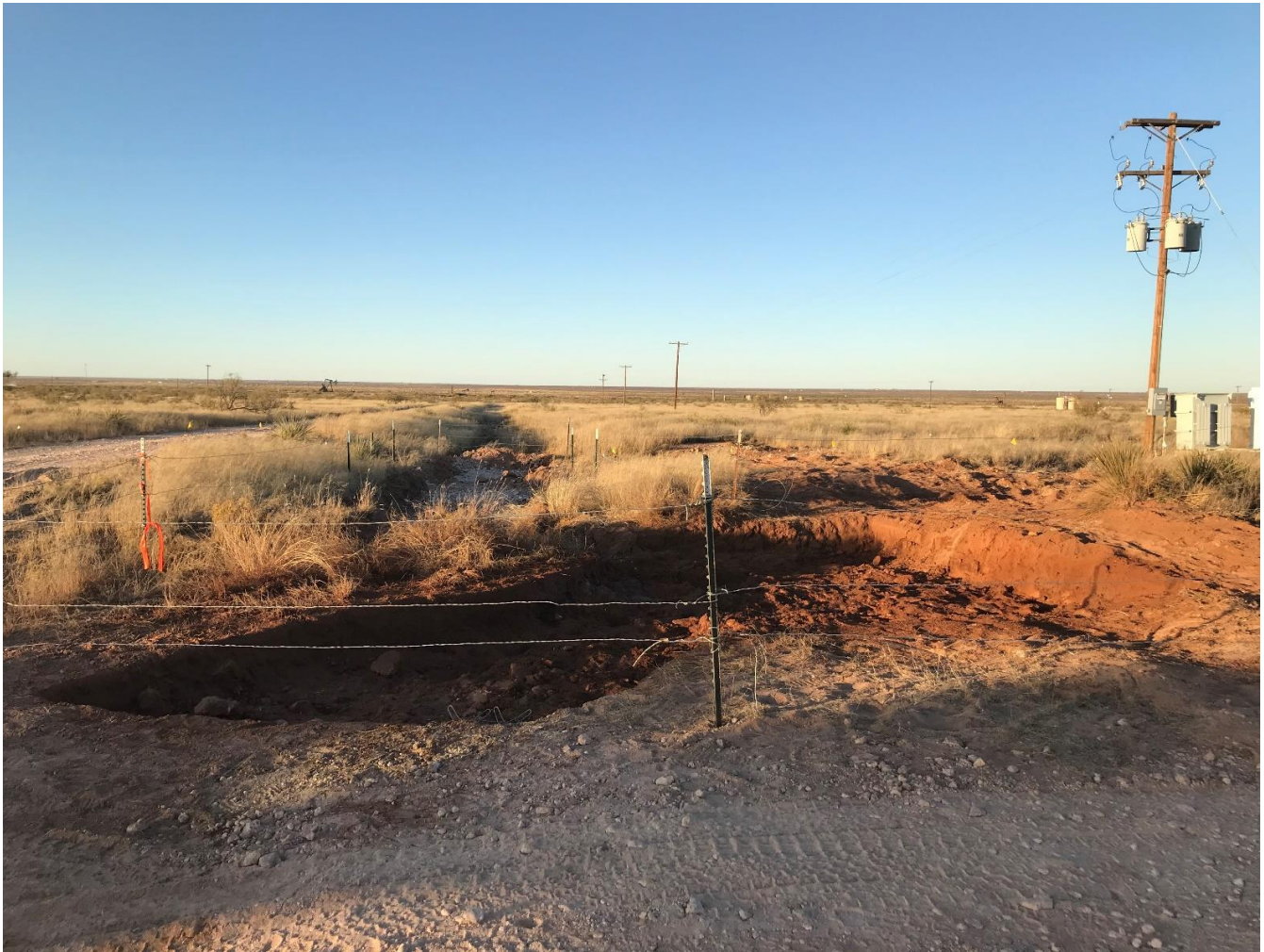
Northern view of final excavation extent in the pasture area during confirmation soil sampling activities.
