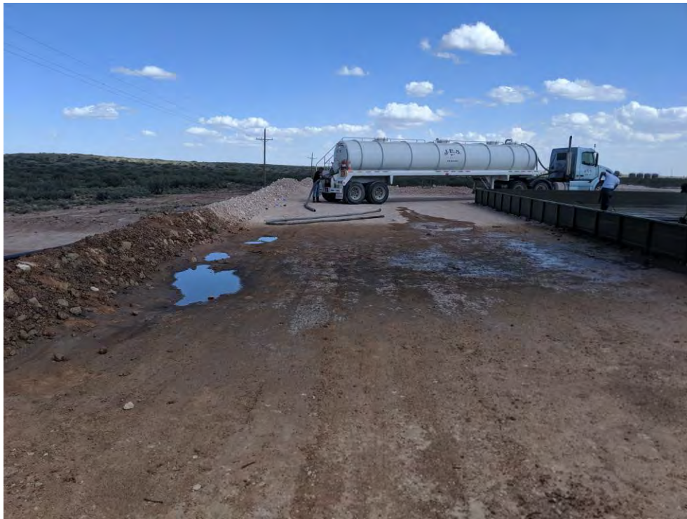
Figure 1: Recovery of released produced water and oil. Photograph is viewing east. The area between the containment wall and north berm of the production pad defines the north/south extent of sampling grid S1 (Plate 1). Date/Time: 2019-10-18 14:01:32. GPS: 32.4584722 N, 103.6010361 W
