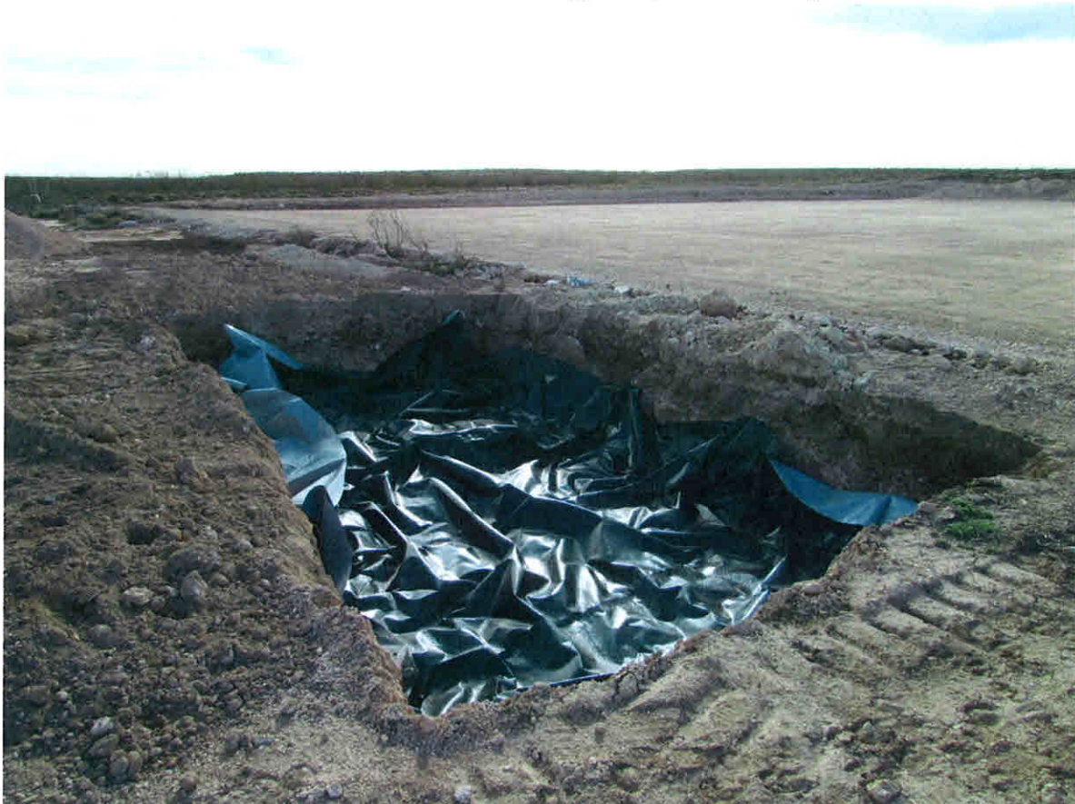
Liner Installed at DP-08-01 Viewing Southwest, December 13, 2016
