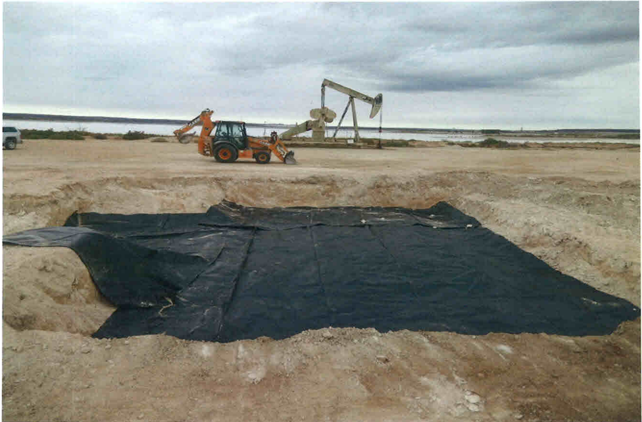
Liner Installed in DP-04-02 (4 feet) Viewing North, November 28, 2016
