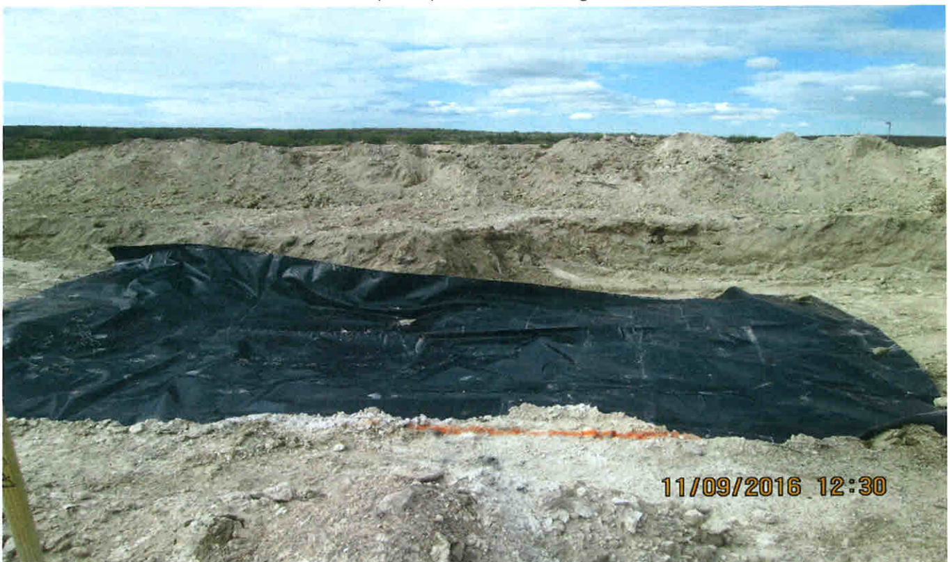
Liner Installed in Excavation (4 feet) DP-05-04 Viewing West, November 9, 2016
