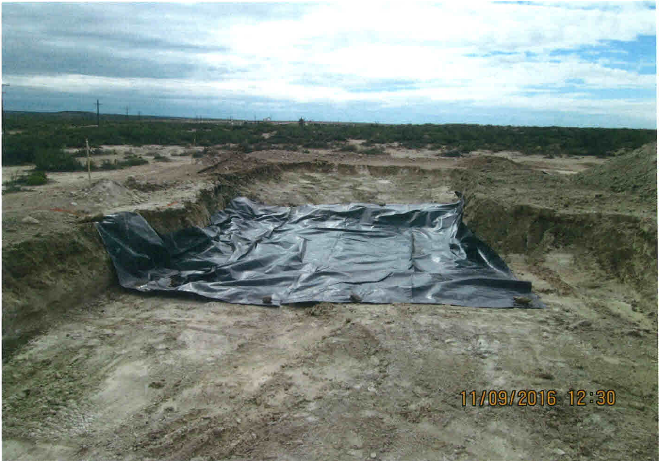
Liner Installed in Excavation (4 feet) DP-05-04 Viewing South, November 9, 2016
