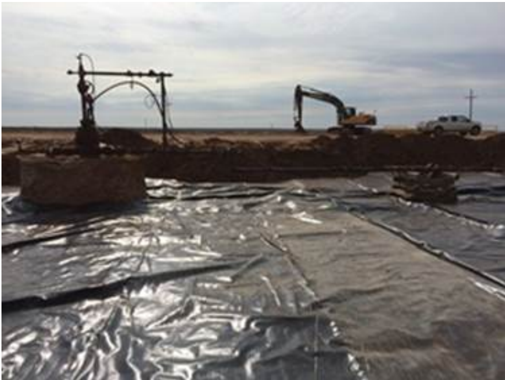
Photograph #6 – Liner installation during remediation of previous release
