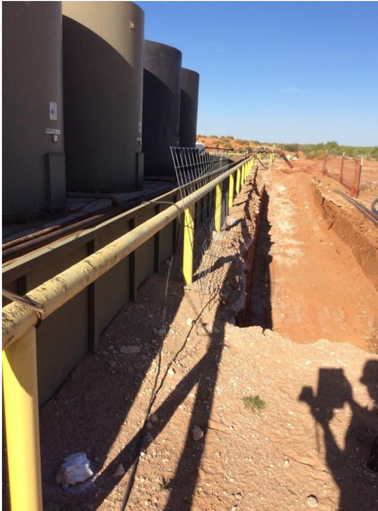
Eastern view of the northern excavation extent during excavation activities.
