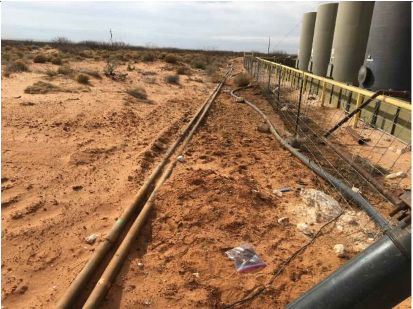
Western view of the soil impacts on pad (right side of center gas lines) and off pad on pasture (left of center gas lines) during delineation activities.
