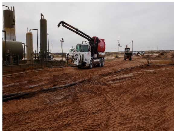
Hydro-vac around gas lines at battery
