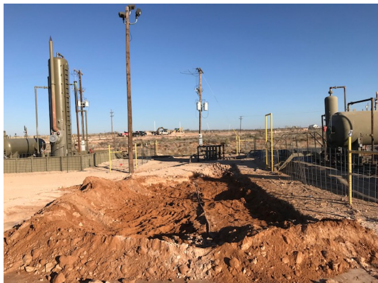
Photograph 3: East facing view of excavation north of process equipment.
