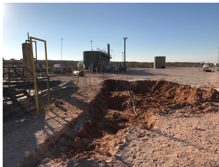
Photograph 2: West facing view of excavation north of process equipment.
