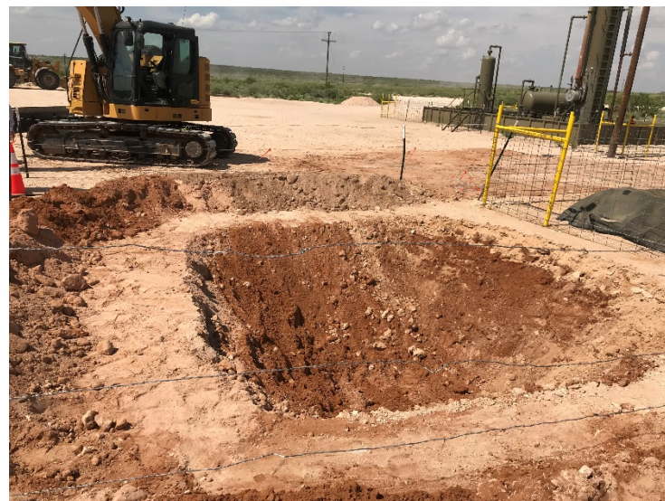
Photograph 4: North facing view of excavation west of process equipment.
