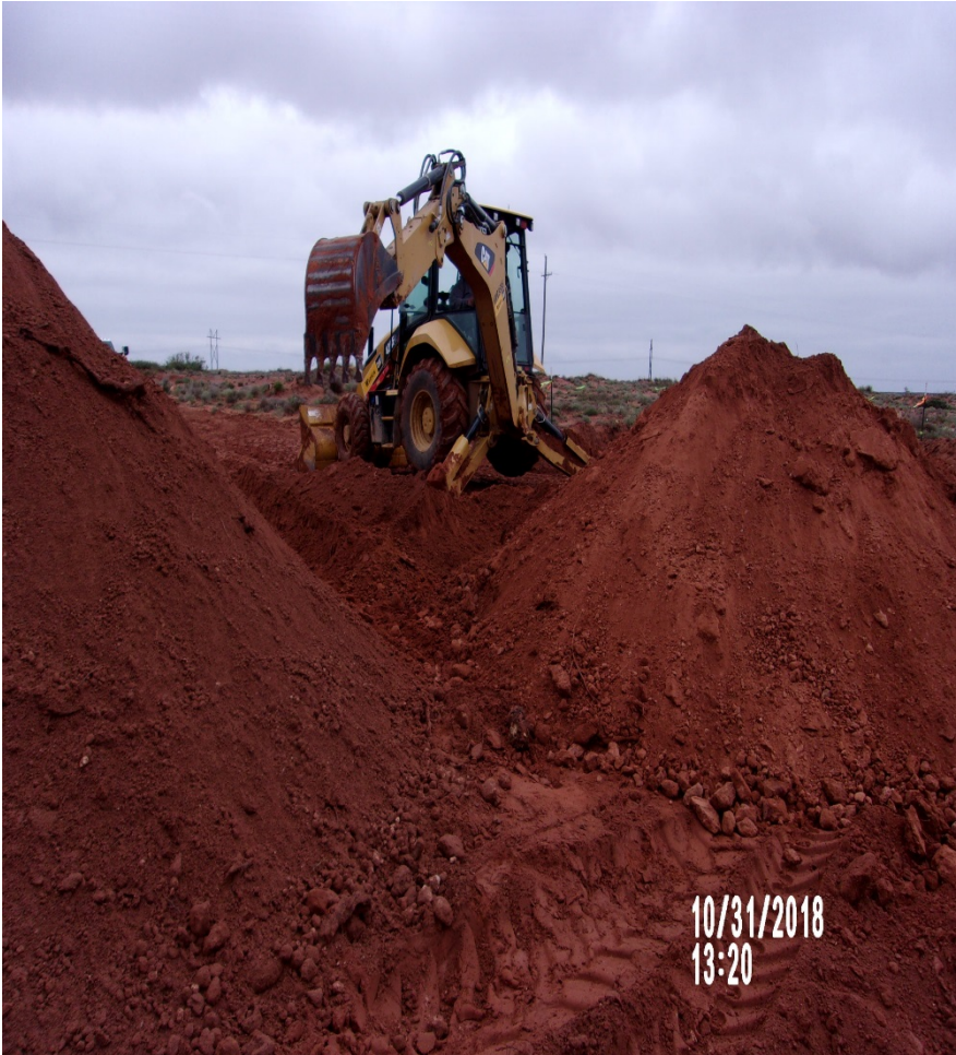
View West – Soil blending of existing stockpiles ongoing.
