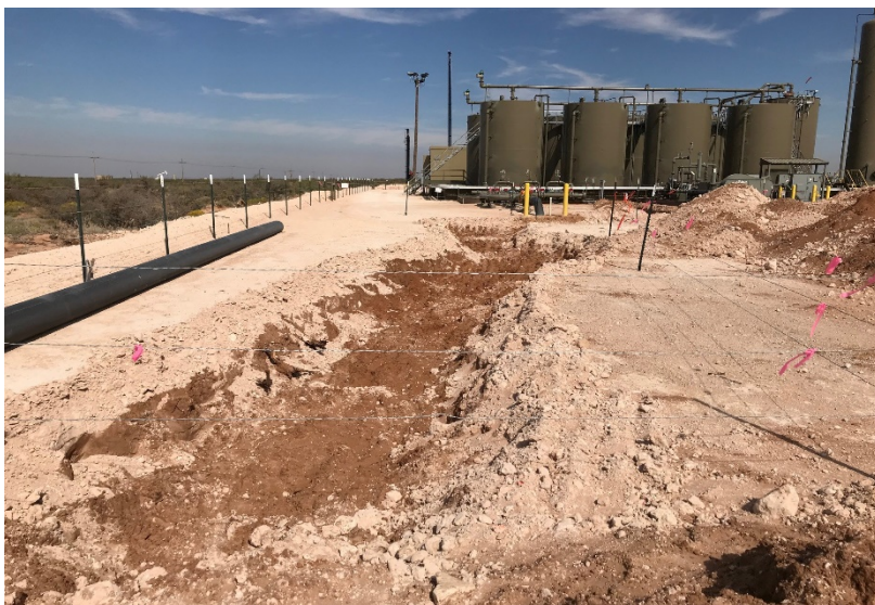
Photograph 3: View of southern end of excavation facing north.
