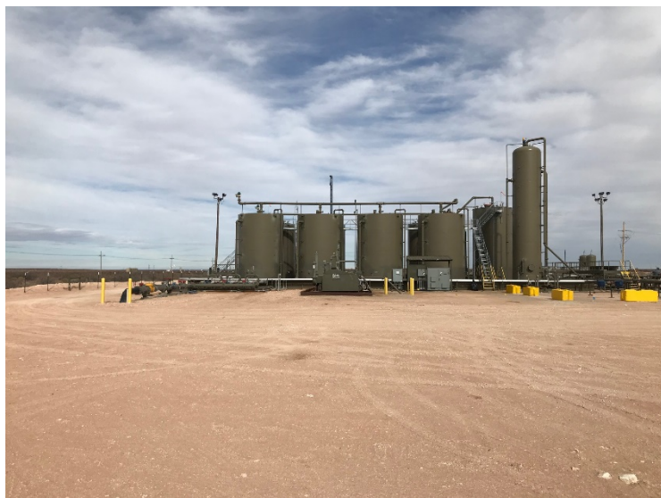
Photograph 1: View of Site and above ground equipment facing north.
