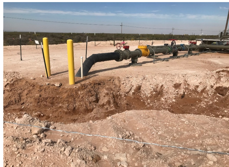
Photograph 4: View of above ground equipment and excavation facing northwest.
