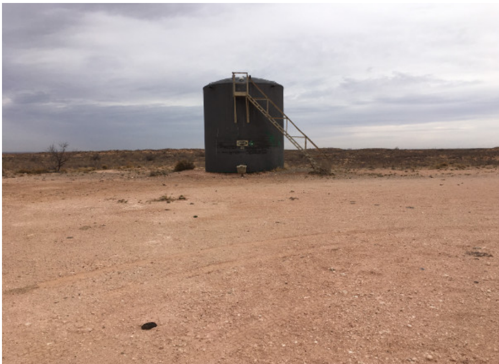
Photograph 1: View northeast of produced water tank.
