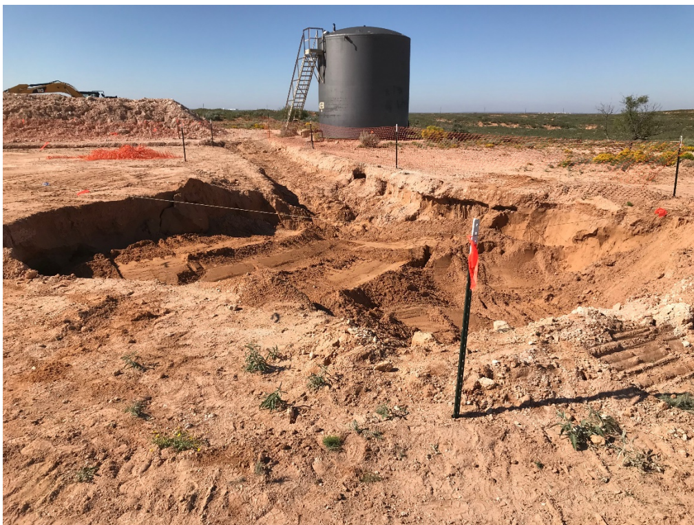
Photograph 2: View south of excavation.
