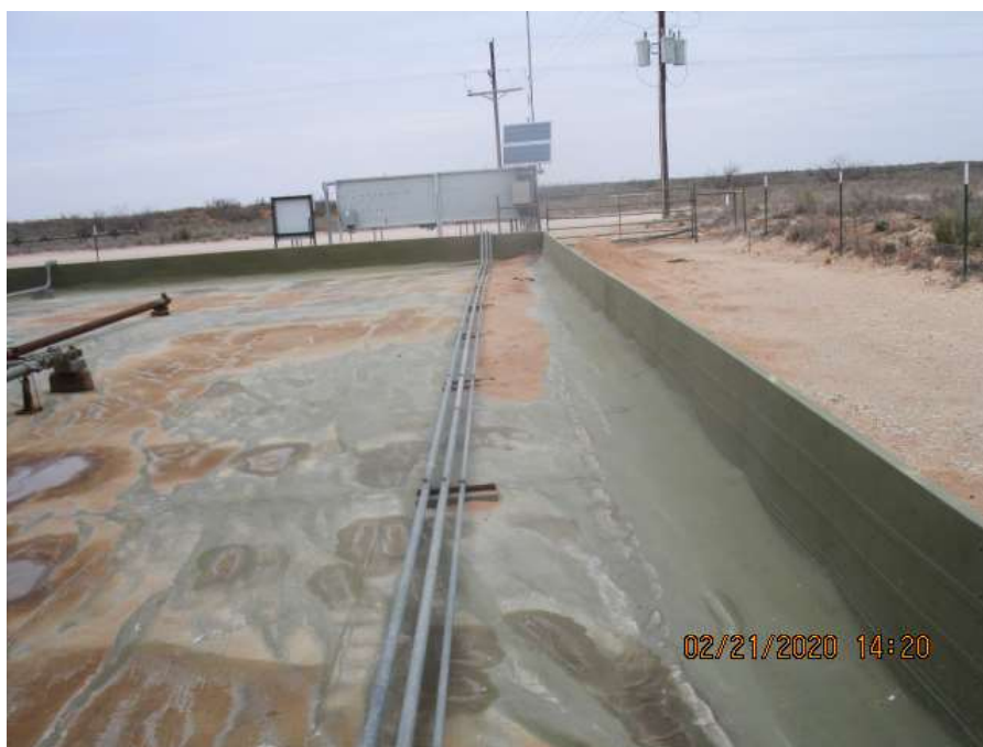
View of sediment and minor pooling within lined secondary containment
