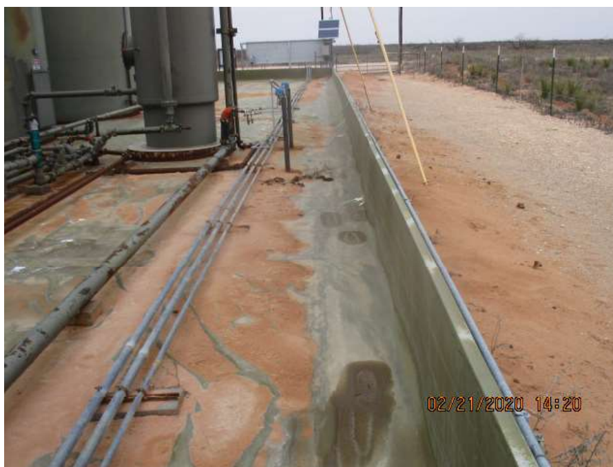
View of sediment buildup within lined secondary containment
