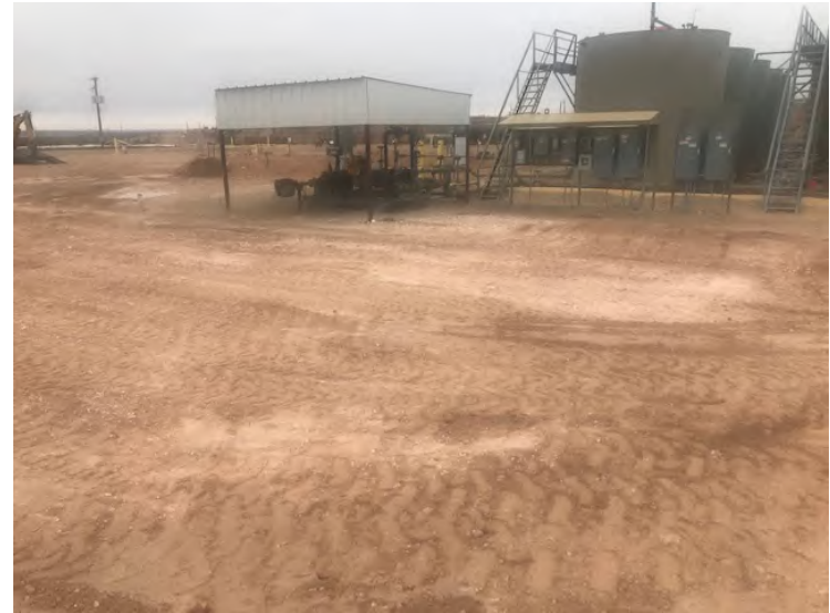
Photograph 4: East facing view of the backfilled excavation.
