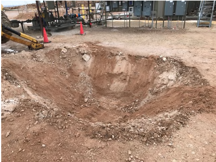
Photograph 3: East facing view of open excavation west of the tanks.
