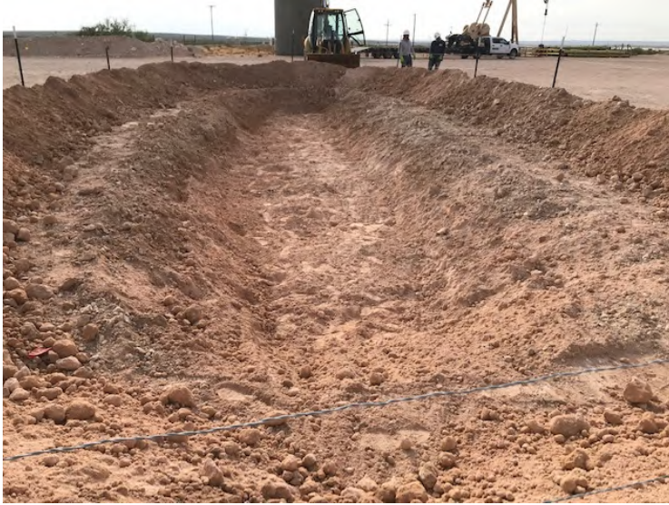
Photograph 1: West facing view of open excavation north of the tanks.
