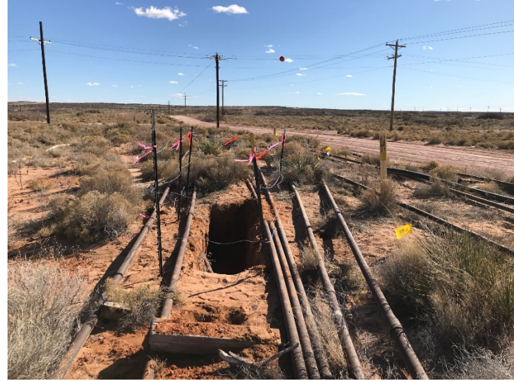
Photograph 2: Southeast facing view of the excavation.
