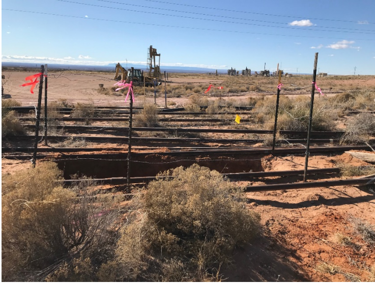
Photograph 1: South facing view of the excavation.
