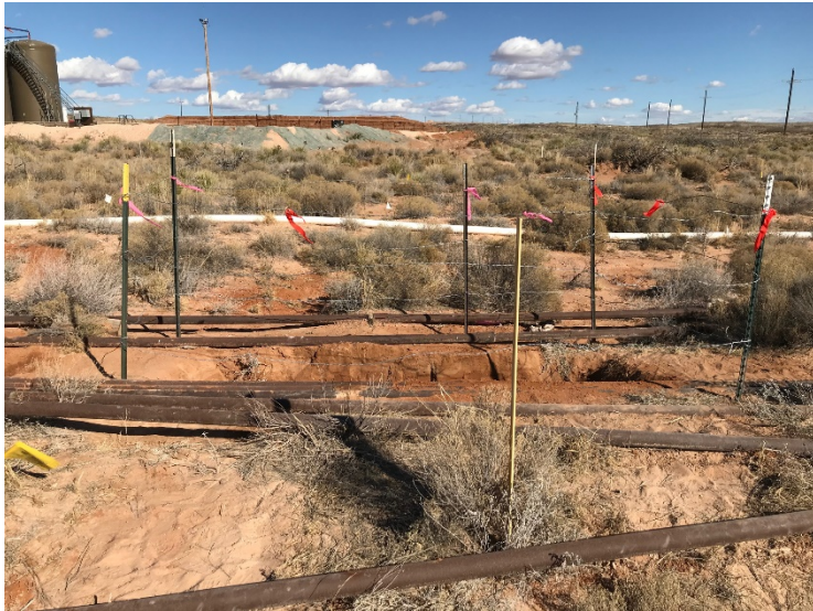
Photograph 3: North facing view of the excavation.
