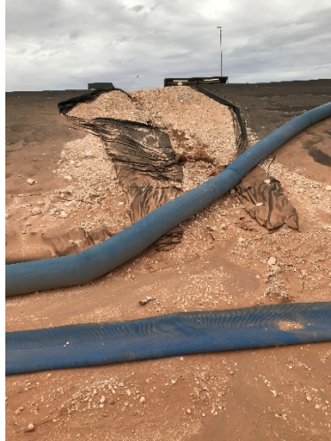
Photograph 1: View of hole in containment lining on east side of Frac Pond.
