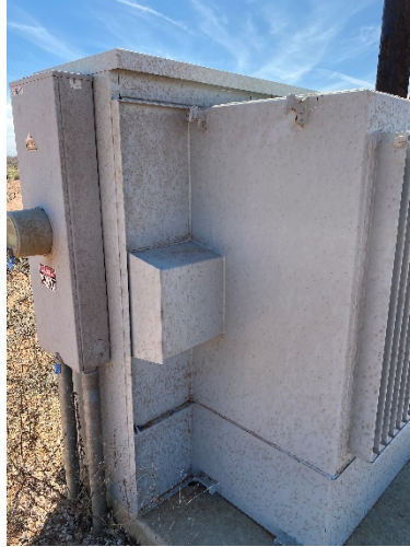
Photograph 1: View of misting from flare on electric box facing southwest.
