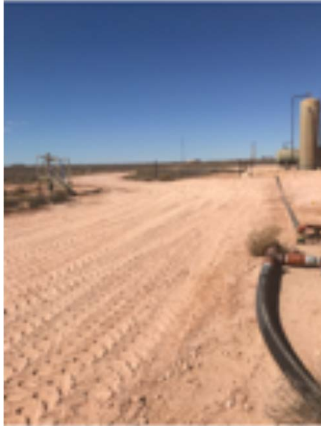
View of Pad Backfilling
