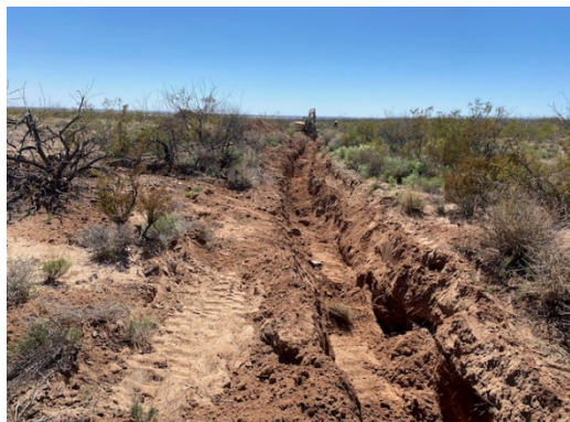
Photograph 17: View of excavation in dry wash facing South.
