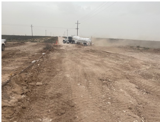
Photograph 14: View of excavation along lease road.
