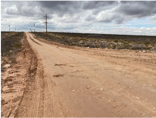
Photograph 1: View of release along lease road.
