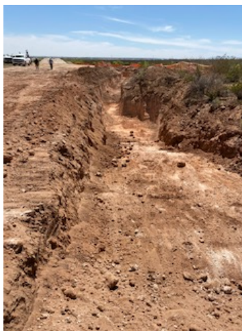
Photograph 16: View of excavation in dry wash.
