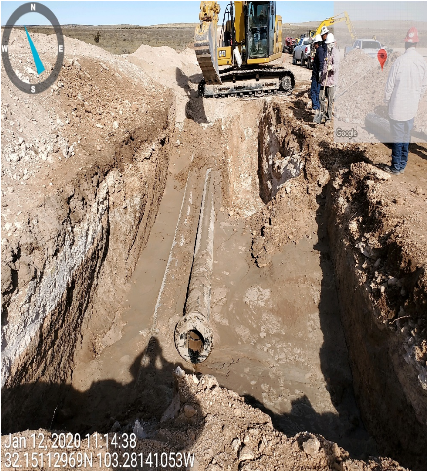
View Northwest – Origin of spill. Release caused by an underground line strike.
