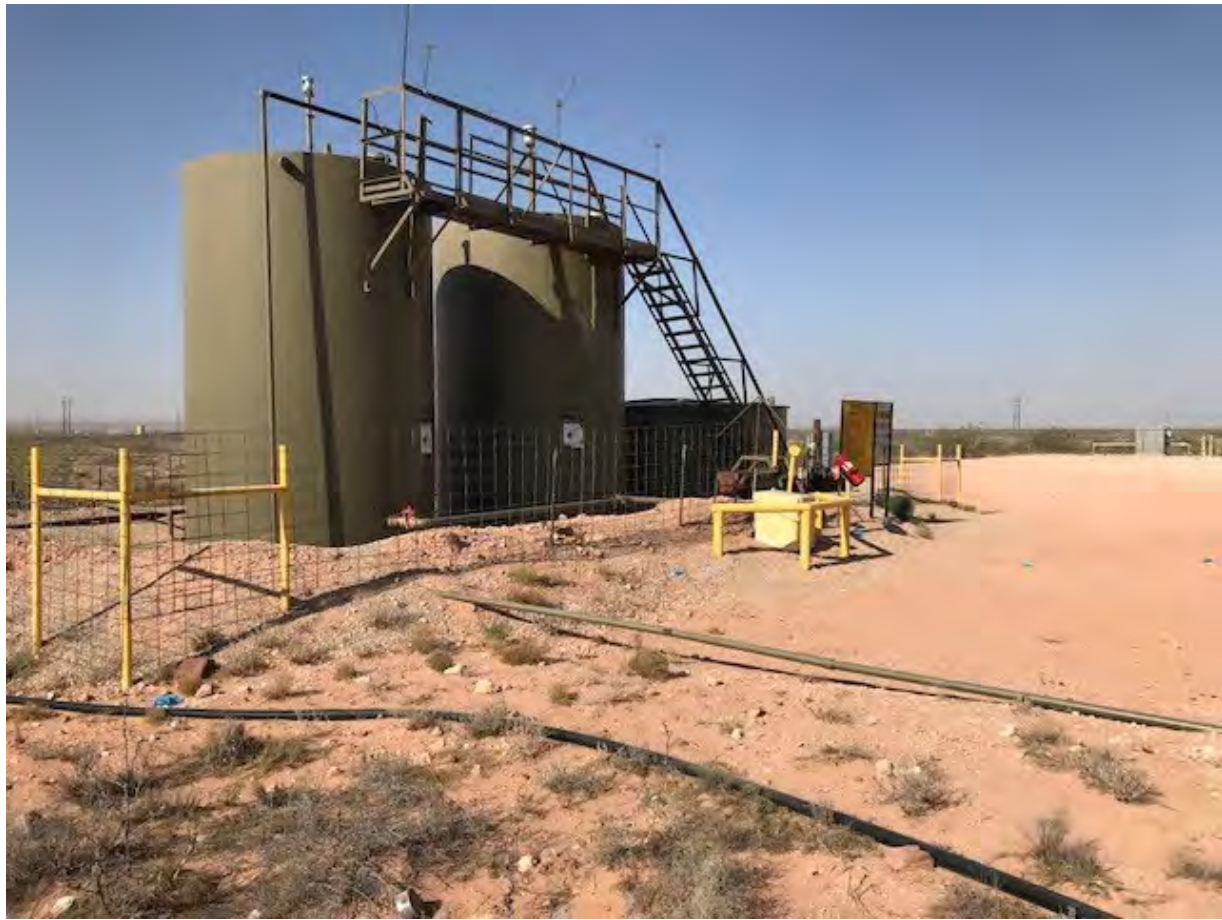
Former James Ranch Unit #10 tank battery location
