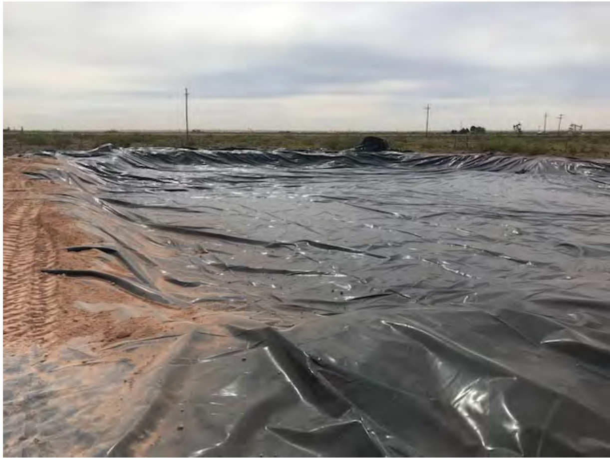
Installation of 30-mil poly liner over excavation extent
