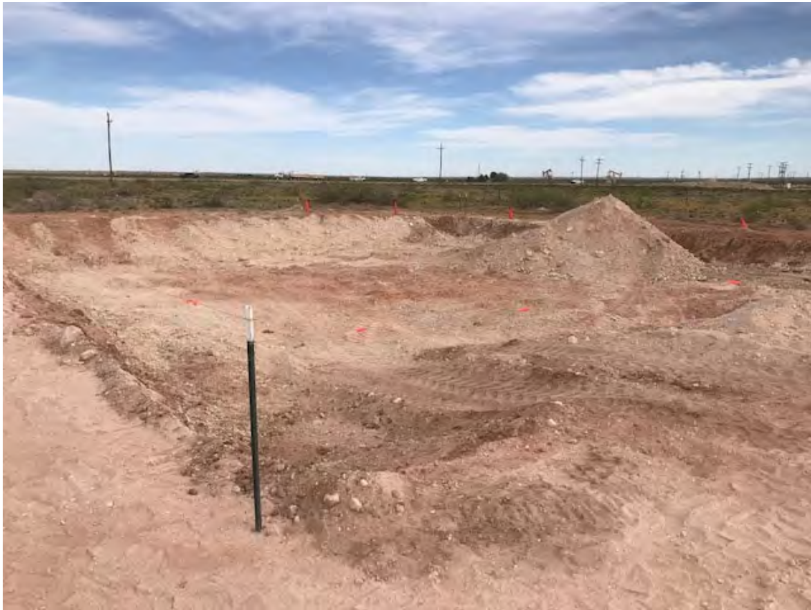
View of open excavation
