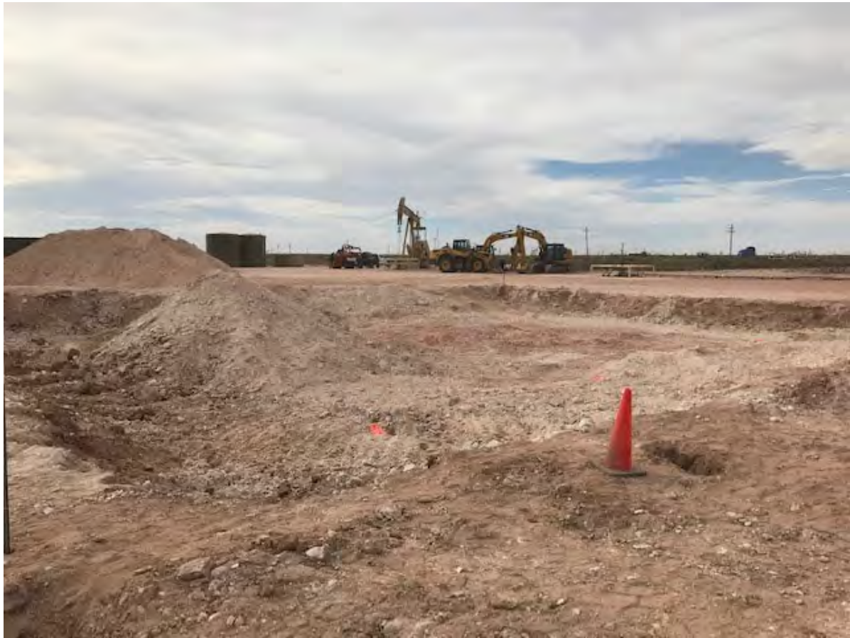
View of open excavation
