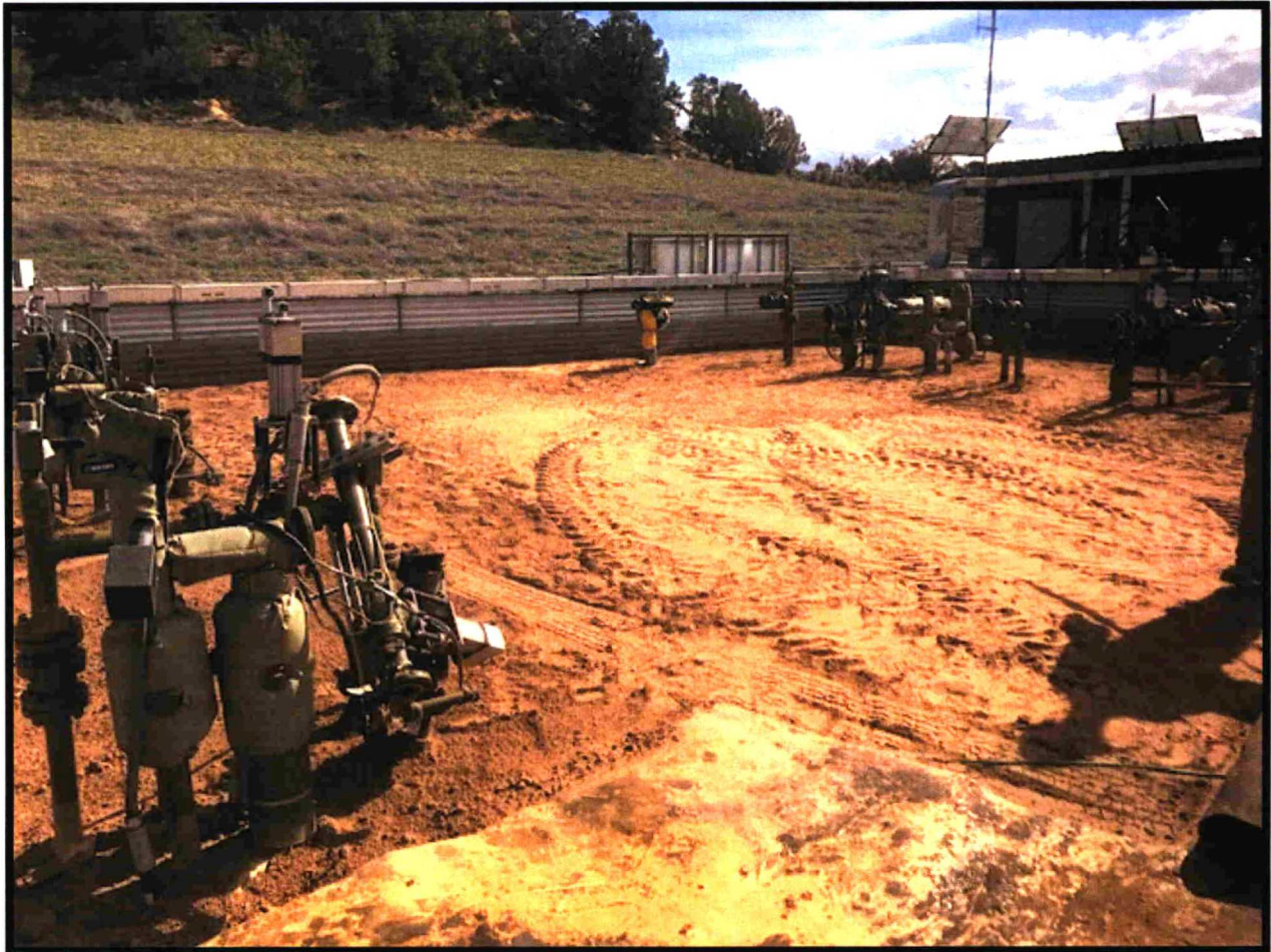
Photo: Area Back Filled
