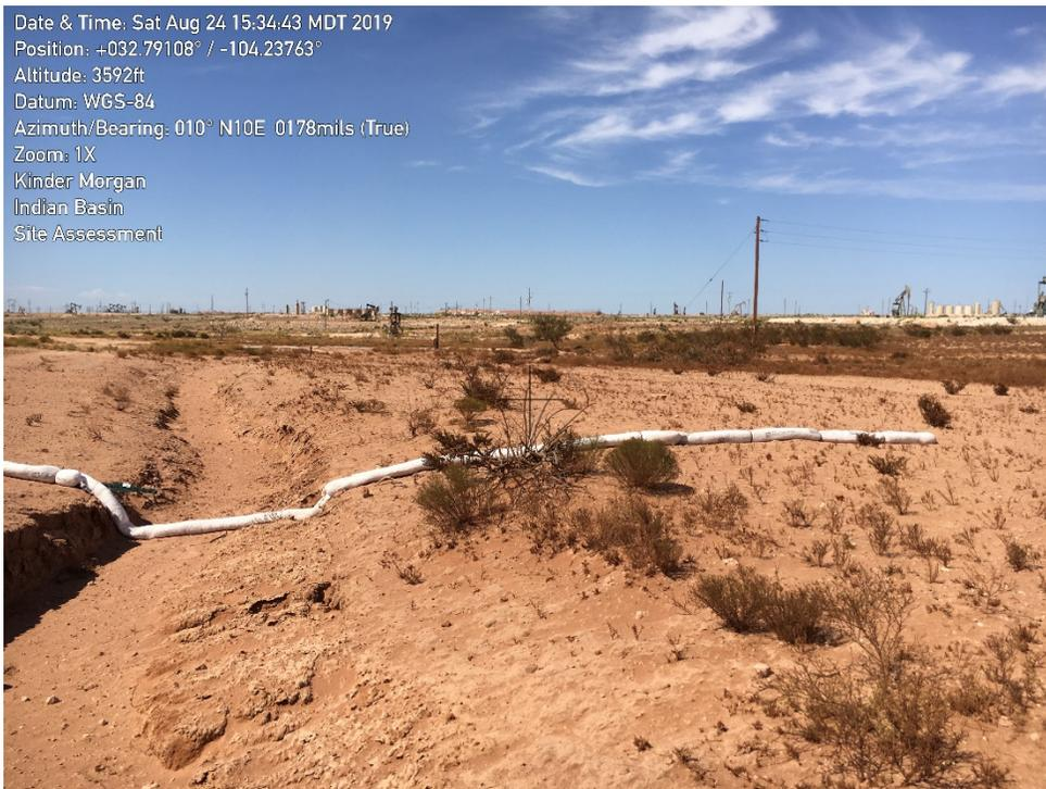
Photo 8. North view of southern-most boom across drainage path.
