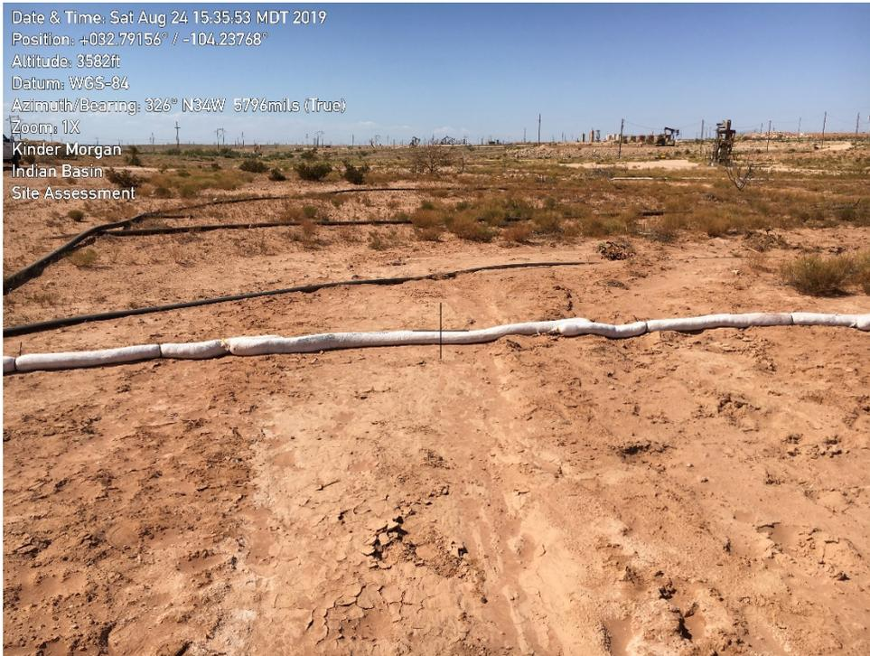
Photo 9. North view of middle boom across drainage path.
