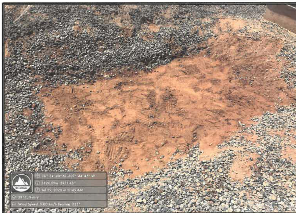
PHOTO 2: Former BGT Location after Removal and Excavation of 6" (7/29/2020)
