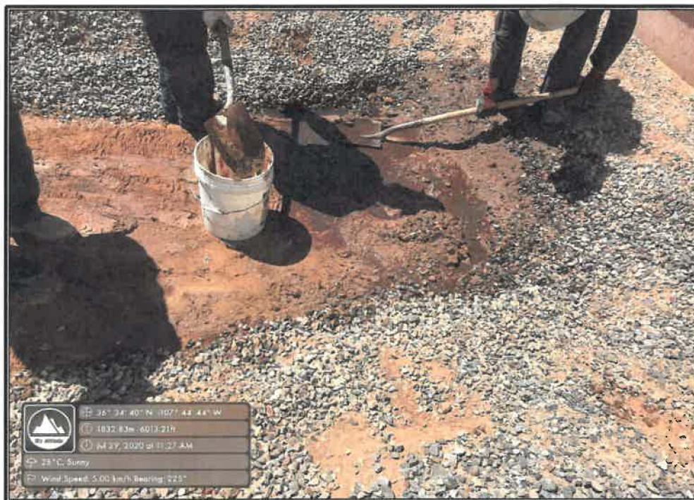
PHOTO 1: Visual Confirmation of Release Occurring During BGT Removal
