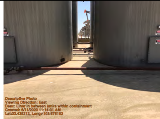
Liner in between tanks within containment
