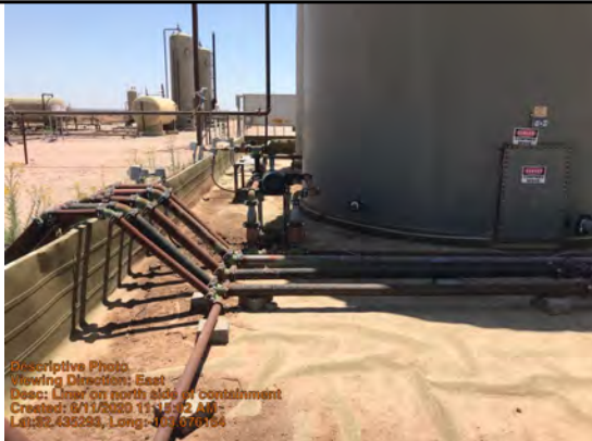
Liner on north side of containment
