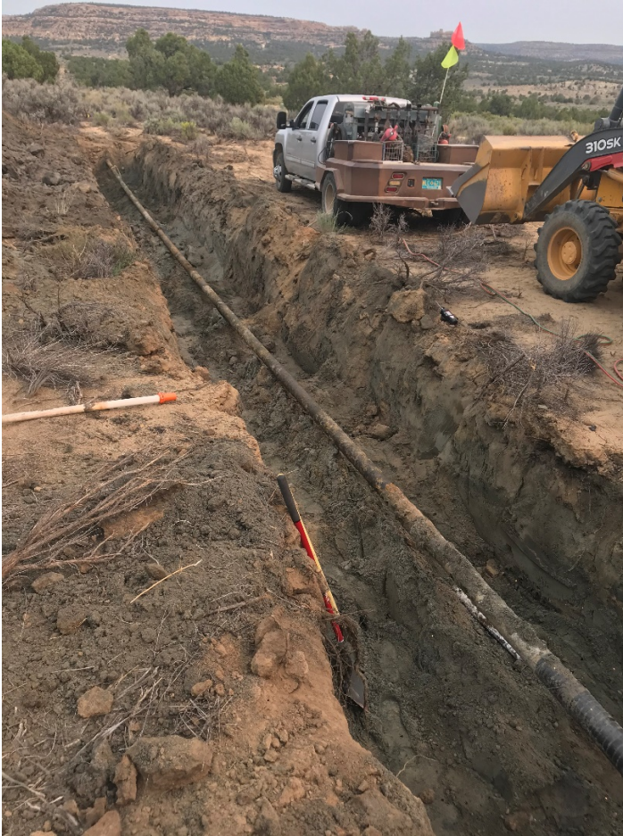
Photo 1: Excavation Around 4-Inch Pipe.
