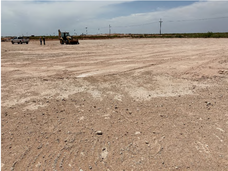
Photograph 5: View of completed backfill on pad.
