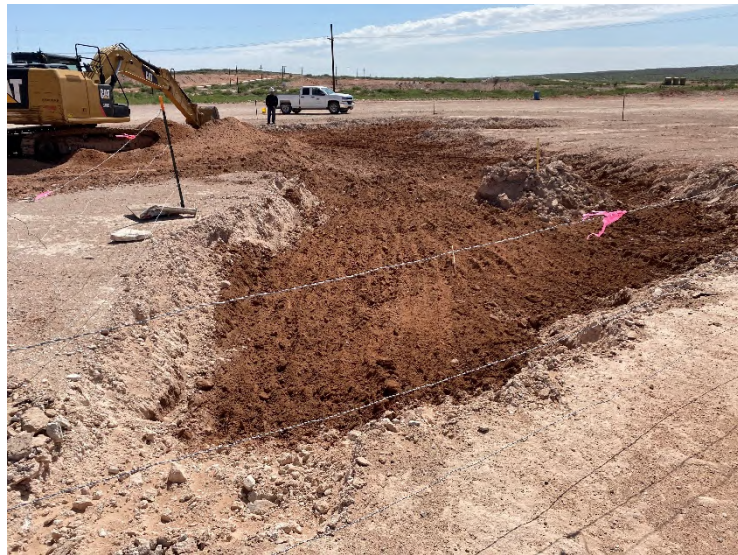
Photograph 3: View of excavation facing southeast.
