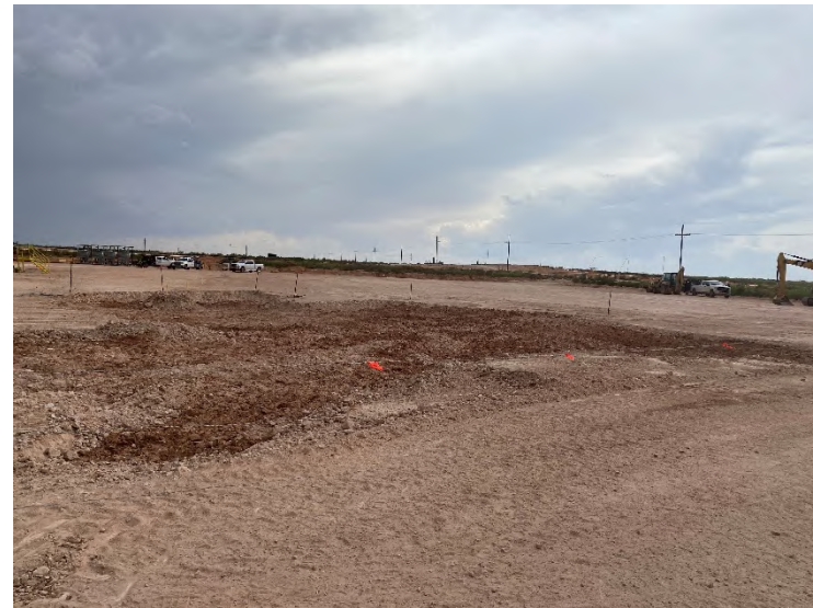
Photograph 4: View of excavation facing northwest.
