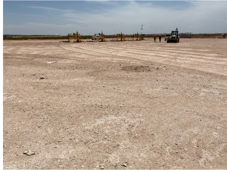
Photograph 6: View of completed backfill on pad.
