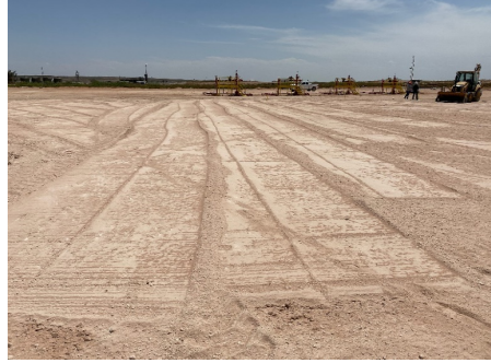
View of backfill on pad completed June 18, 2020. Recontoured and graded to match well pad surface.
